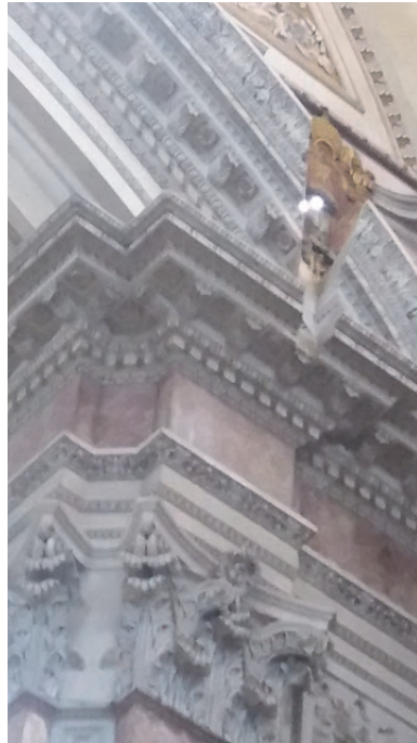
Fig. 2. The cut in Vanvitelli's cornice made in order to let the light from the gnomon reach the meridian line. The photo is on April 6, 2019 at 13:19:53. The two luminous points are the pinhole and, lower, the light reflected by the carved marble of the frieze.
