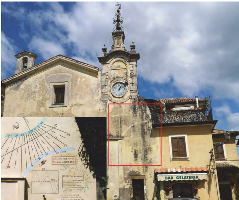
Fig. 5. Sundial of Angelo Secchi in Boville Ernica (FR) as in April 2019 and when restored in 1996; the gnomon is parallel to the polar axis, the analemma and the equation of time vanished. 7 This sundial was restored in 1950 by the astronomer Giuseppe Armellini, buried in the nearby Church's crypt, and again by Nicola Severino in 1996. 8 Now it deserves another restauration as it is evidenced with the rectangle. In the left low side its status in 1996.
