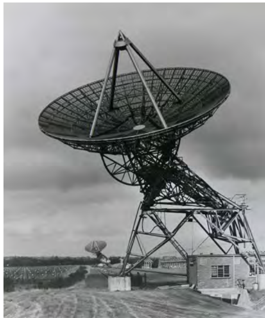
Fig. 2. The Cambridge One-Mile Telescope, the world's first fully-steerable, general purpose, Earth-rotation aperture synthesis radio telescope.
