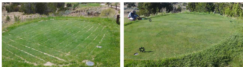
Figure 5 Example of tee boxes 1 month after subsurface drip irrigation (SDI) installation. Left: trench lines were dug directly into the turf canopy and rootzone. Right: sod was removed, SDI was installed by trenching only into the rootzone and sod was returned in place.
