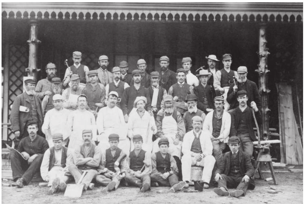
Figure 5.1 Craftsmen working on Mar Lodge, Aberdeenshire, c.1910. © National Museums Scotland.
