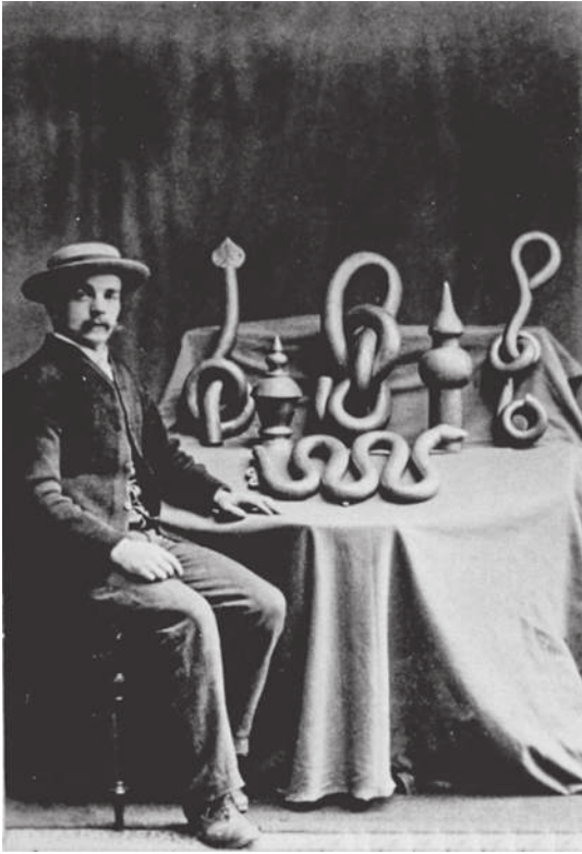
Figure 6.2 T. M. Ross, plumber of Haddington. Exhibition display of pipework, c.1886. © East Lothian Council Archives – Jack Tully Jackson Collection.
