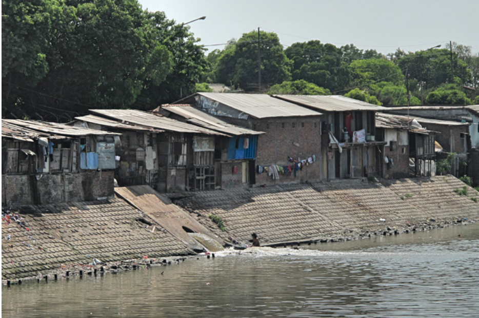
Fig. 51 The houses of Kampung Baru formed at the northern levee of Kali Jagir Photo: Christian Obermayr, 2015
