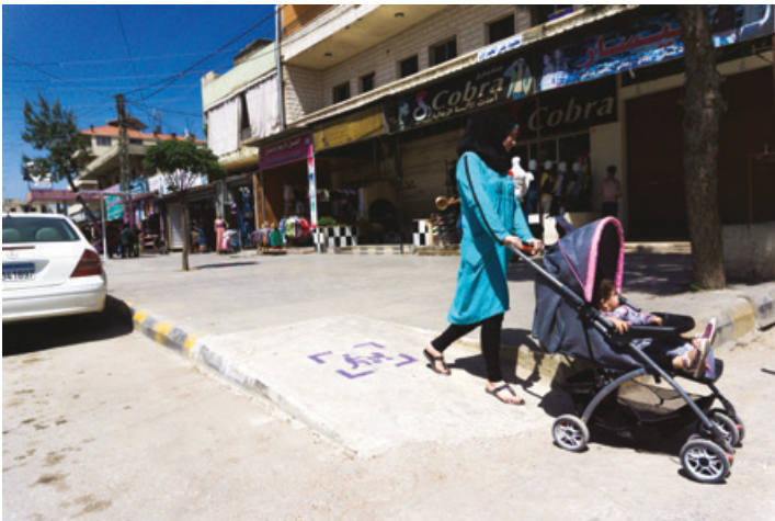
Figure 5.4 Access ramp onto high pavement.
