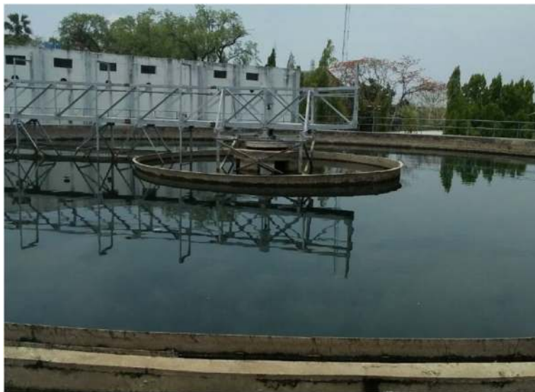
Figure 2.10 Sedimentation tank in water treatment plant (courtesy of Nagpur Municipal Corporation and Orange City Water Private Limited, India).
