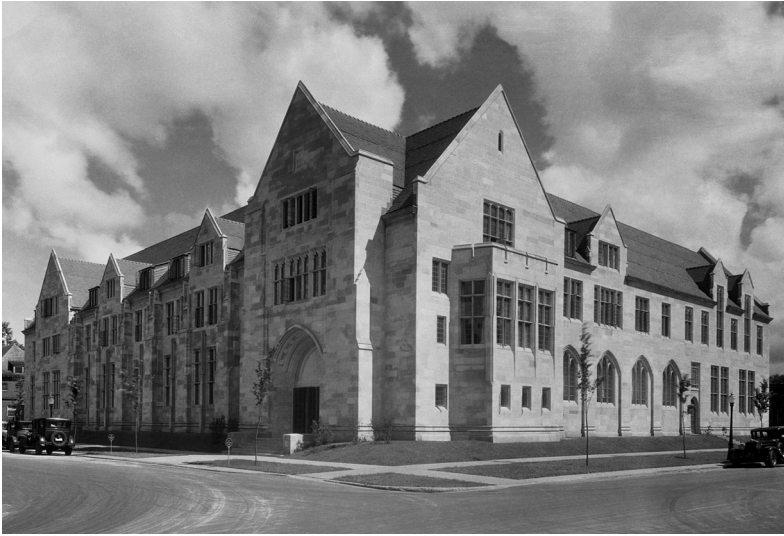
Figure 4.6 Oriental Institute building from the northwest, designed by Oscar Harold Murray and completed in 1931, ca. 1931, P. 18730/N. 10872. Source: Courtesy of the Oriental Institute of the University of Chicago. Reproduced under a CC BY-NC-ND 4.0 licence.
