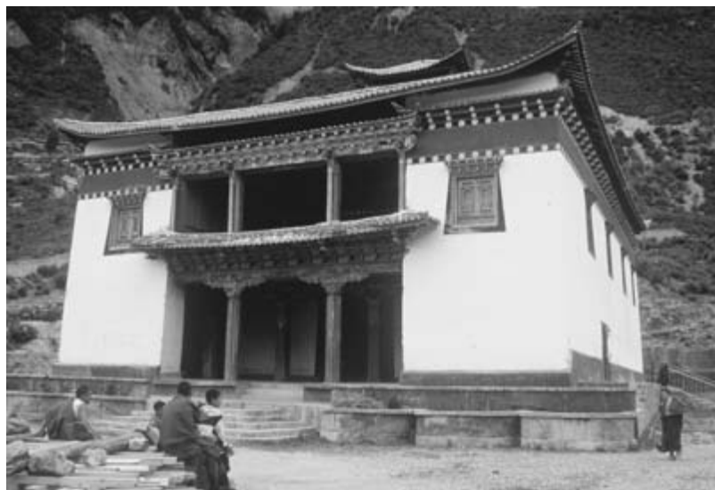
FIG. 2.1. The Assembly Hall of Dechenling Monastery in Dechen County was still under construction at the time of our visit in 1998. Adjacent to the monastery was a small boarding school where all subjects were taught in Tibetan.
