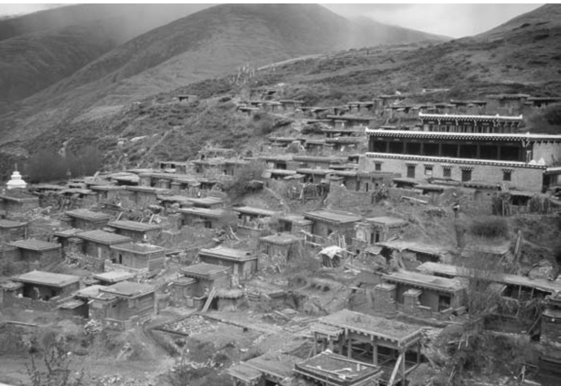
FIG. 2.2. A nunnery in Kandze. The nuns were working hard to build new living quarters.
