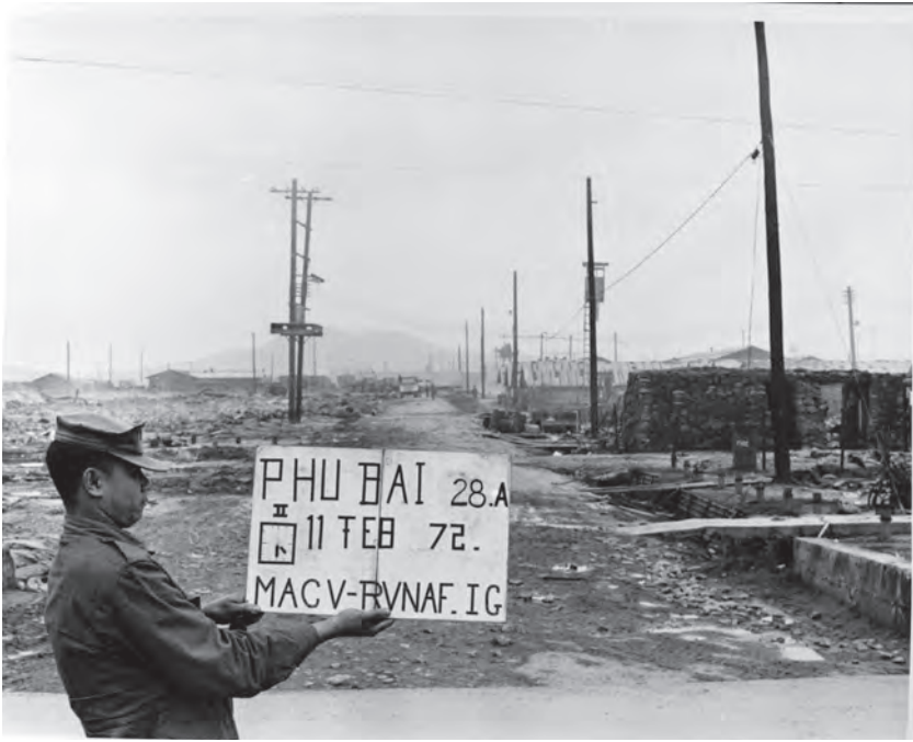
FIGURE I.1. Demolished troop billets at Phú Bài Combat Base, February 11, 1972. Source: Box 3, RVNAF Base Turnover Inspections, MACV Inspector General Records, Record Group 472, US National Archives and Records Administration, College Park.
