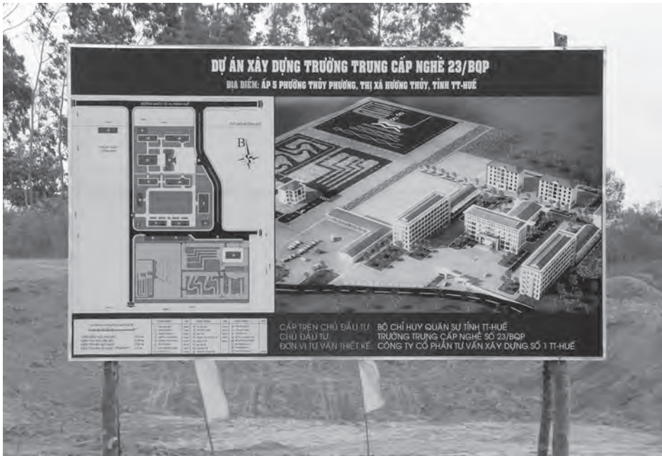
FIGURE 6.4. Construction site for Vocational College 23 on top of the former 160th Aviation Group site. Photo by author, July 2015.
