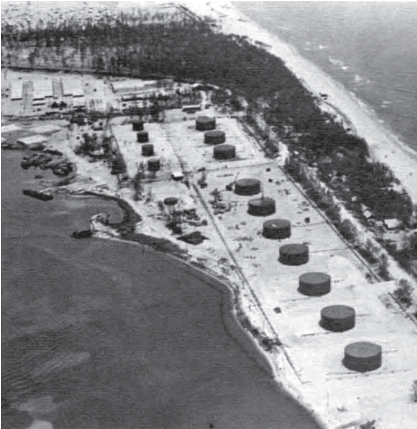
FIGURE 5.6. Reconstructed petroleum-oil-lubricant tank farms near Thuận An. Source: US Navy Mobile Construction Battalion Eight, MCB 8: Hue, Phu Bai, 1968 (Minneapolis: American Yearbook Company, Military Division, 1968), 9.
