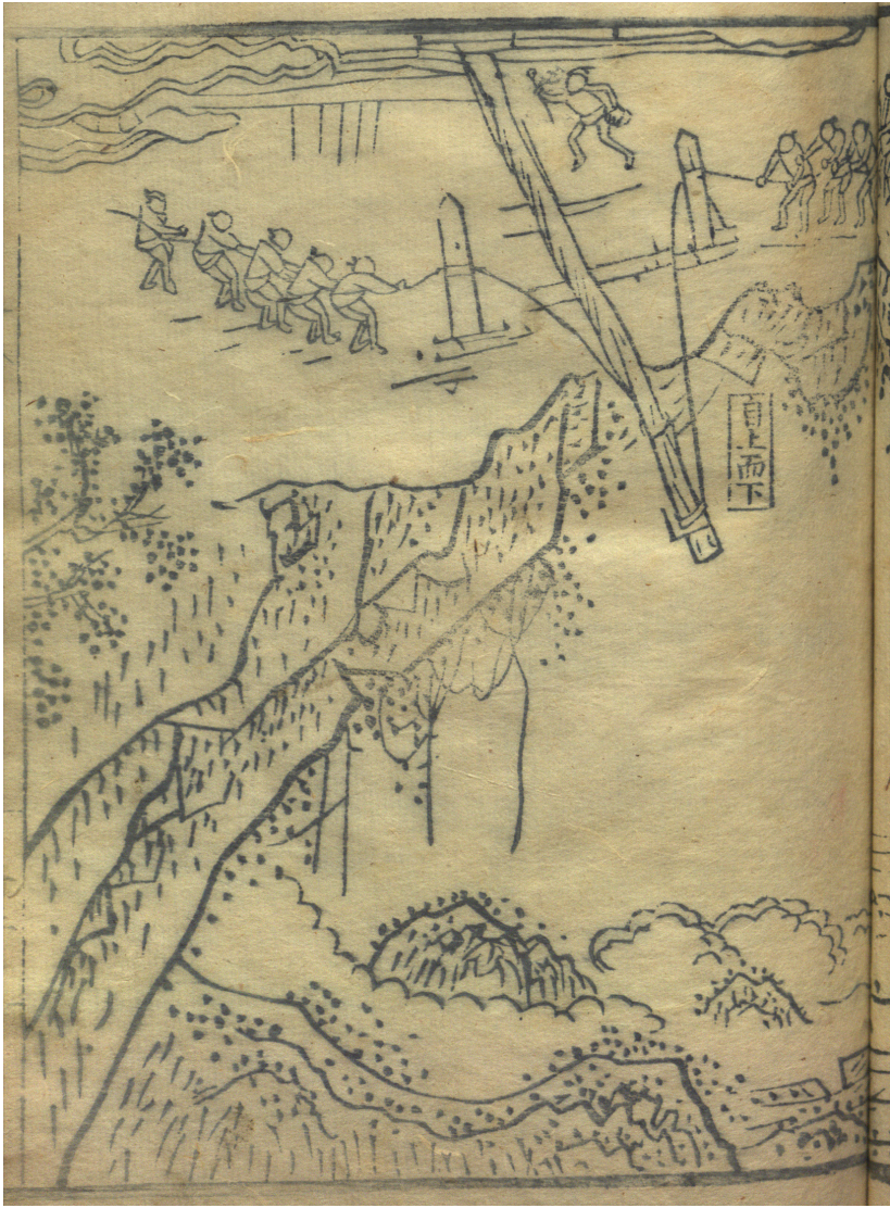
FIG 7.1 Lowering logs off a cliff. Detail of a woodcut from Essays on Timber Rafting in the Western Regions (Xi cha huicao; 1533). Courtesy of the Library of Congress, Chinese Rare Book Digital Collection.
