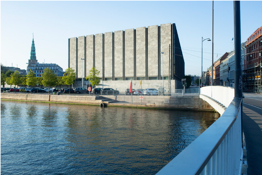
Figure 9.1: Exterior of the National Bank, Copenhagen (© Jens Frederiksen)
