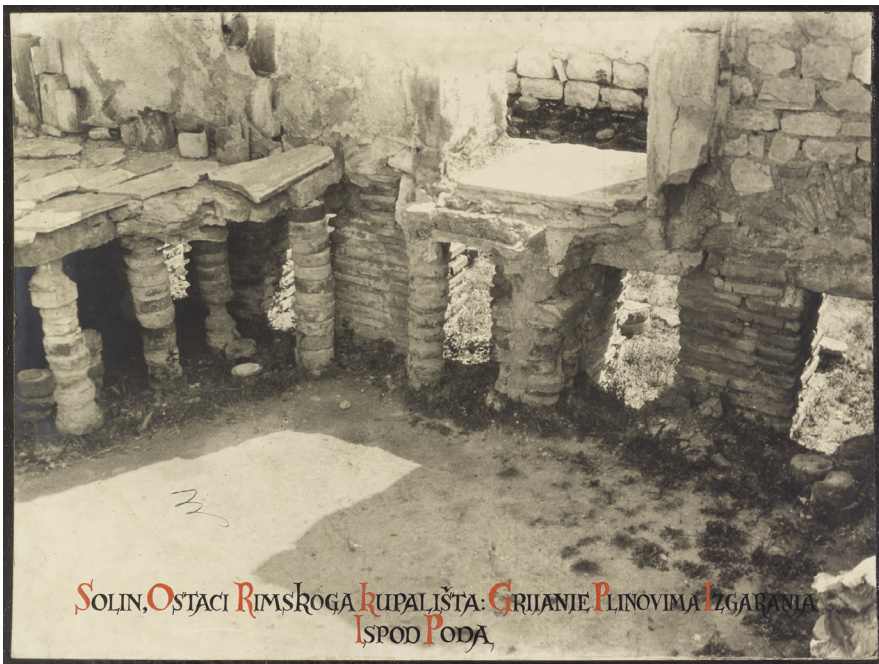
Figure 6.1: Solin, remnants of a Roman bathhouse: underfloor heating by gases. (Croatian Museum of Medicine and Pharmacy, Croatian Academy of Sciences and Arts, HMMF-2464)
