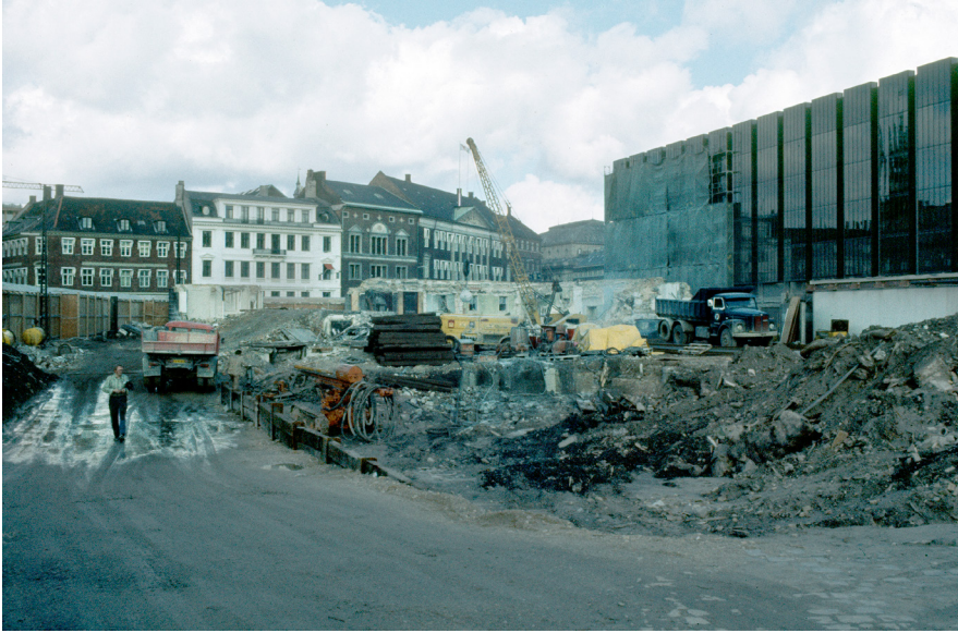
Figure 9.3: Demolition of the National Bank, Copenhagen (© Jens Frederiksen)
