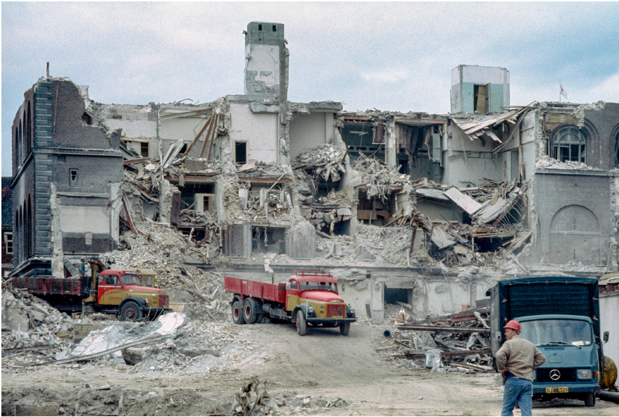
Figure 9.4: Demolition of the National Bank, Copenhagen (© Jens Frederiksen)
