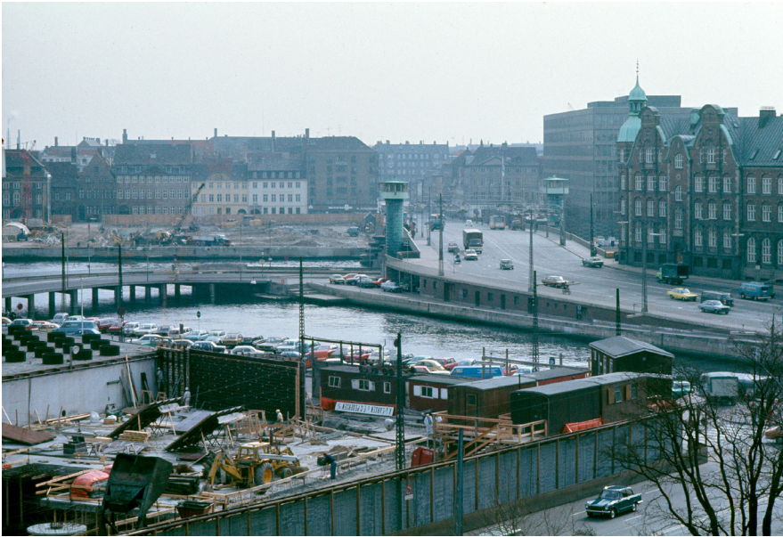
Figure 9.2: Construction site of the National Bank, Copenhagen (© Jens Frederiksen)
