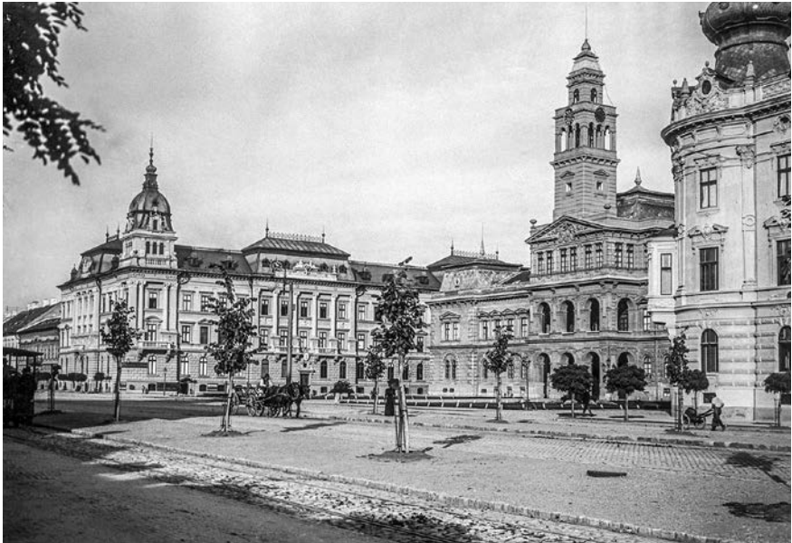
Figure 7.10. Arad, Andrassy Square with the city hall, 1901. Source: Fortepan, 27255, Frigyes Schoch.
