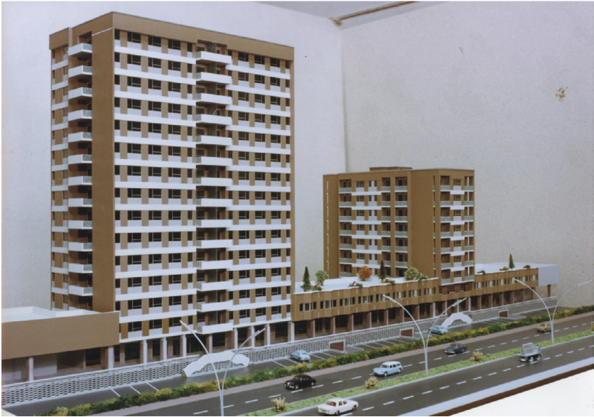
Figure 6.5: Maquette of the 15-storey tower and the 8-storey building connected by a 2-storey continuous slab block with commercial portico and roof gardens, built along the new highway. Model by Enzo Dolci, 1964. Courtesy of Riccardo Carver
