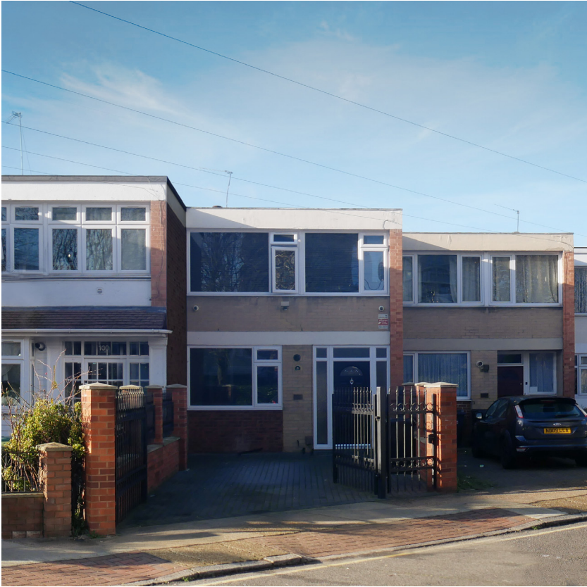
Figure 2.8: LCC housing was later subject to privatisation under Thatcher’s “Right to Buy” policies. Already explicating property boundaries through exposed parti walls, staggered plans, and garden walls, it is still quite easy for buyers to adapt each house without much consequence to the collective form. Lansbury Alton Street Extension, Neighbourhood 9. Photograph by author, 2023
