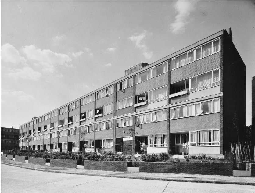
Figure 2.7: Exposed brick parti walls in LCC blocks, which identified the divisions between each maisonette, were often decorative: they were separated from the actual parti wall by a waterproof membrane. Concrete slabs between each maisonette were exposed, while intermediate floors were concealed, further articulating the building as an aggregation of dwelling units. St. Annes (Locksley Street) Estate in Neighbourhood 4a, LCC Photograph Collection. © London Metropolitan Archives (City of London)
