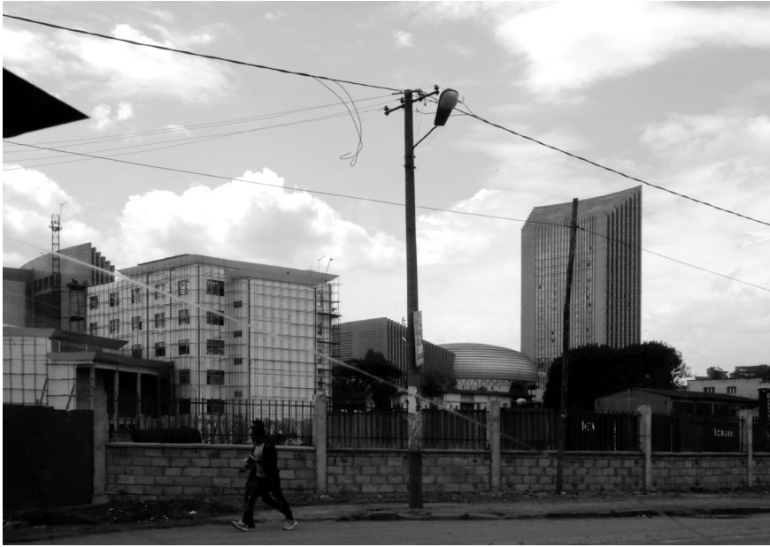
Figure 9.1 View of the AU building from a nearby street (Daniel Mulugeta, March 2019).
