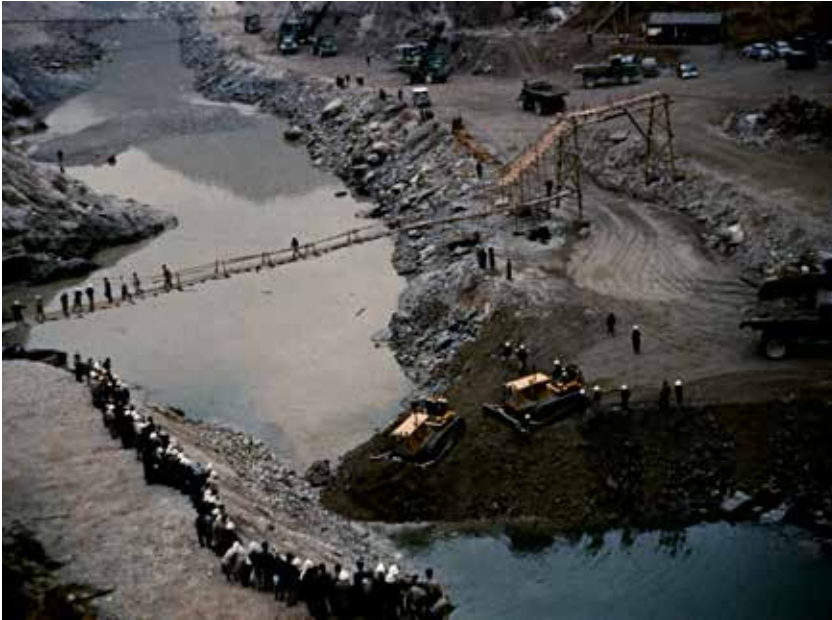
Fig. 8.3. Blocking and diverting the Tenryū River in Sakuma Dam . Picture courtesy Documentary Film Preservation Center, Japan.
