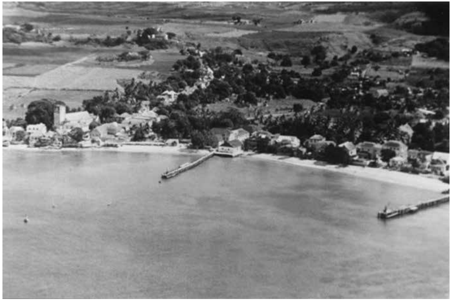
Figure 20.4. Aerial view of (c. 1940s) two (now demolished) jetties at Speightstown; view looking west (courtesy Karl Watson).
