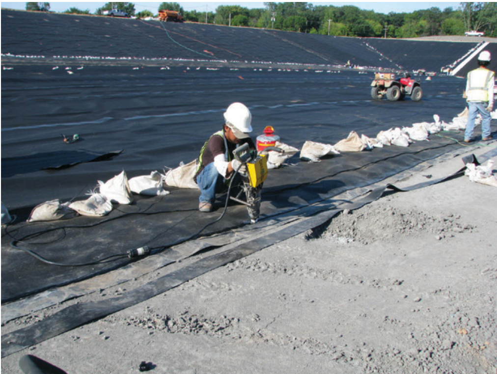
Figure 8.8 A plastic liner (geomembrane) to capture landfill leachate. Image: MPCA Photos.
