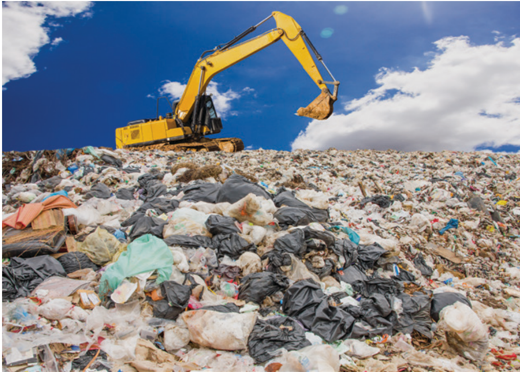
Figure 8.13 Mining of landfilled waste is associated with physical, chemical and biological hazards. Image: Shutterstock.
