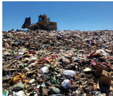
Bulldozer distributing waste at the Gila County landfill, Arizona, United States (Alan Levine).
