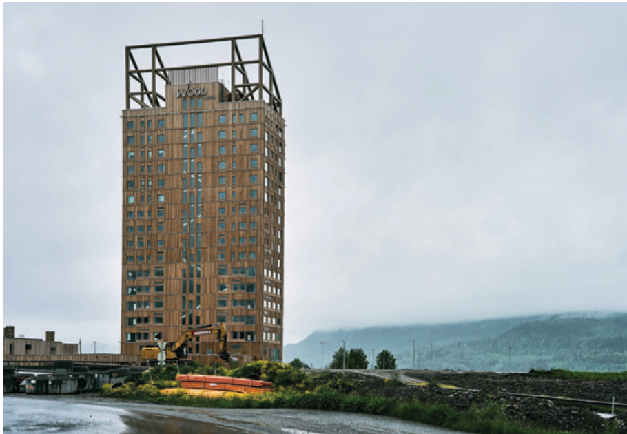
Figure 7.17 This tower in Norway is one of the tallest structures in the world made with CLT. Image: Øyvind Holmstad.
