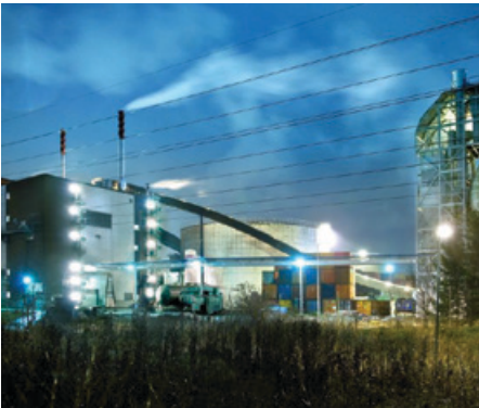
Waste incineration facility producing electricity and district heat, Uppsala, Sweden (Vattenfall).
