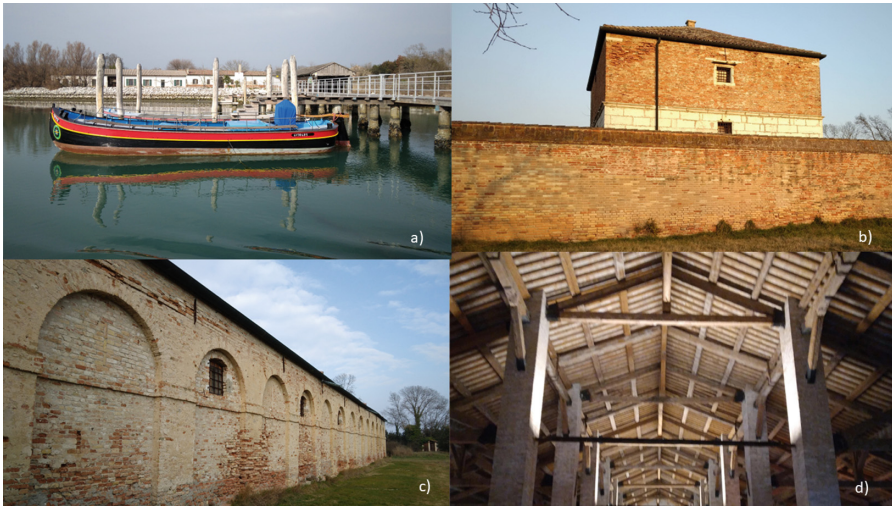
Fig. 1. The Lazzaretto Nuovo Island, a) access pier; b) ancient gunpowder store; c) Tezon Grande, exterior; d) Tezon Grande, interior
