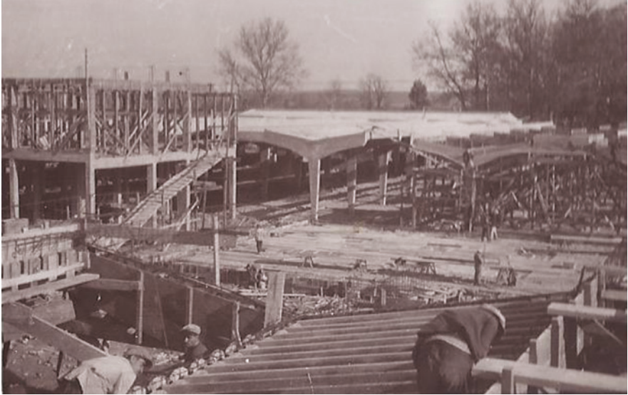
FIGURE 13 Construction site, 1934 COURTESY OF EMRE ÖNCÜ
