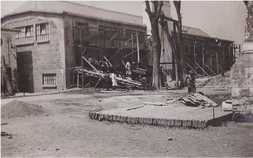
FIGURE 17 The construction of the new production building, 1934 COURTESY OF EMRE ÖNCÜ
