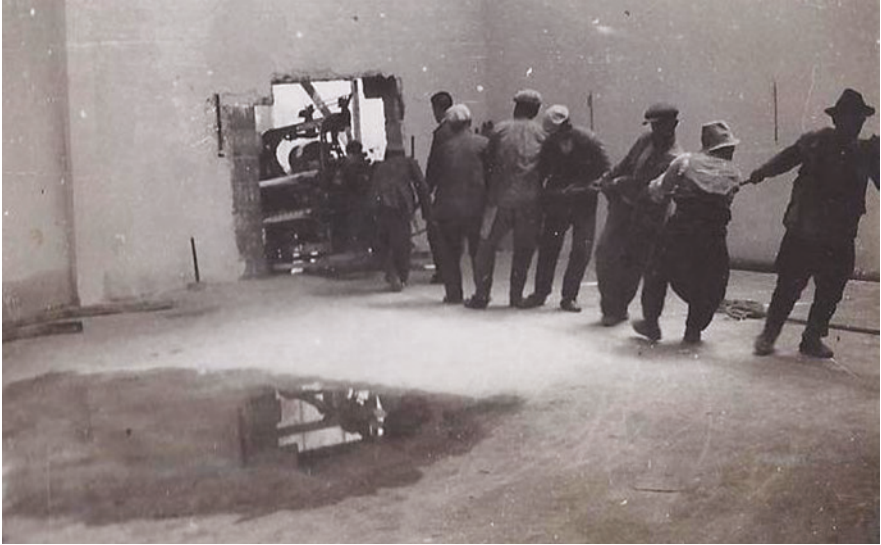
FIGURE 18 Workers bringing in new machinery to the new production building, 1934 COURTESY OF EMRE ÖNCÜ
