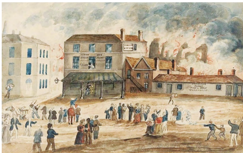
Figure 5. Fire at Albion Wharf and Mill, March 1841.
