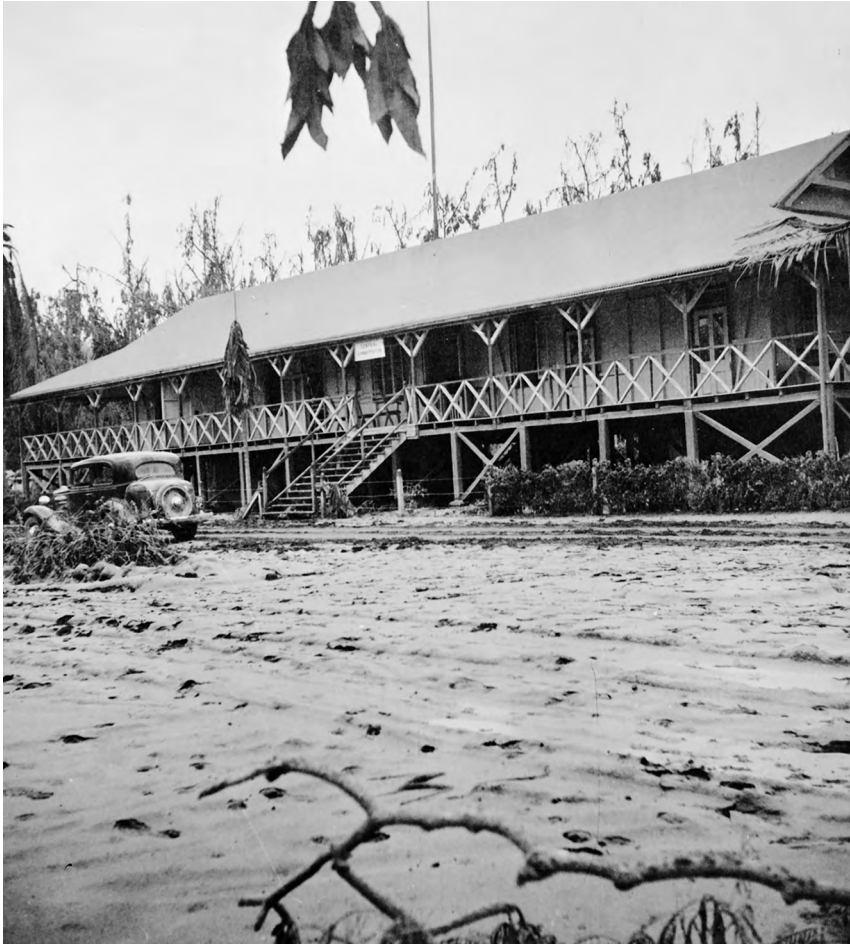
Figure 3.47. Central administration building and ash-covered road.
