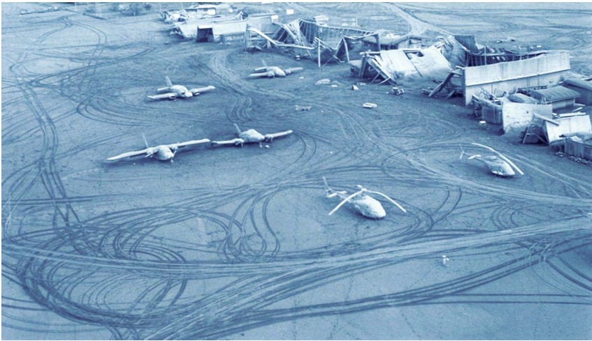
Figure 8.9. Lakunai Airfield damage including ash-covered aircraft.
