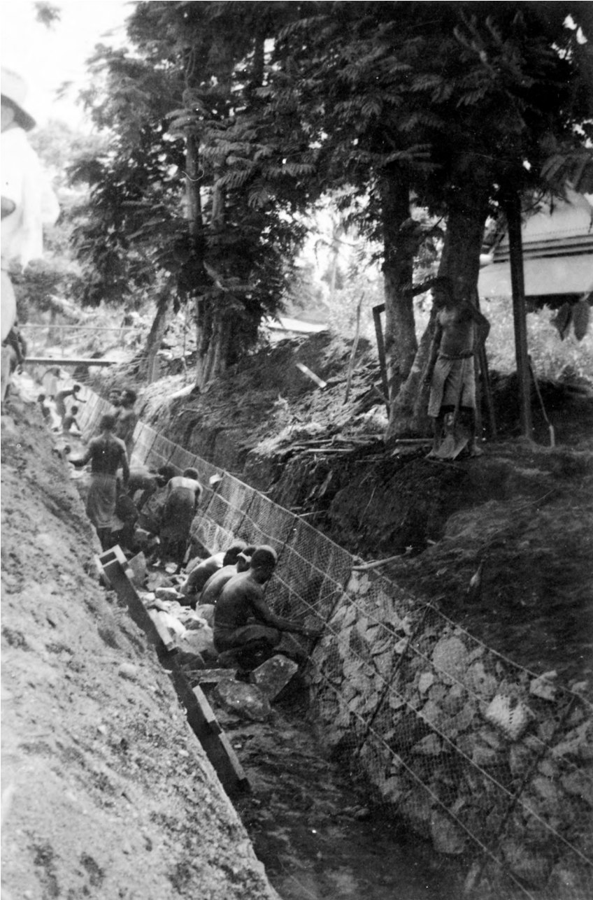
Figure 3.64. Construction of drains in Rabaul.
