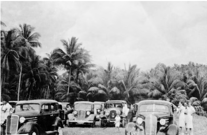
Figure 3.20. Car parking at Nodup after Rabaul evacuation.
