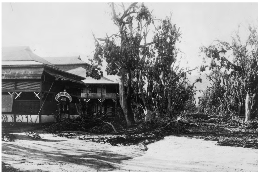
Figure 3.42. Mango Avenue damage.
