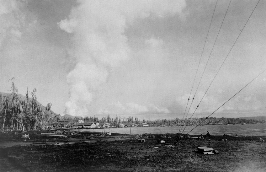
Figure 3.45. Damage along Rabaul frontage near radio station.
