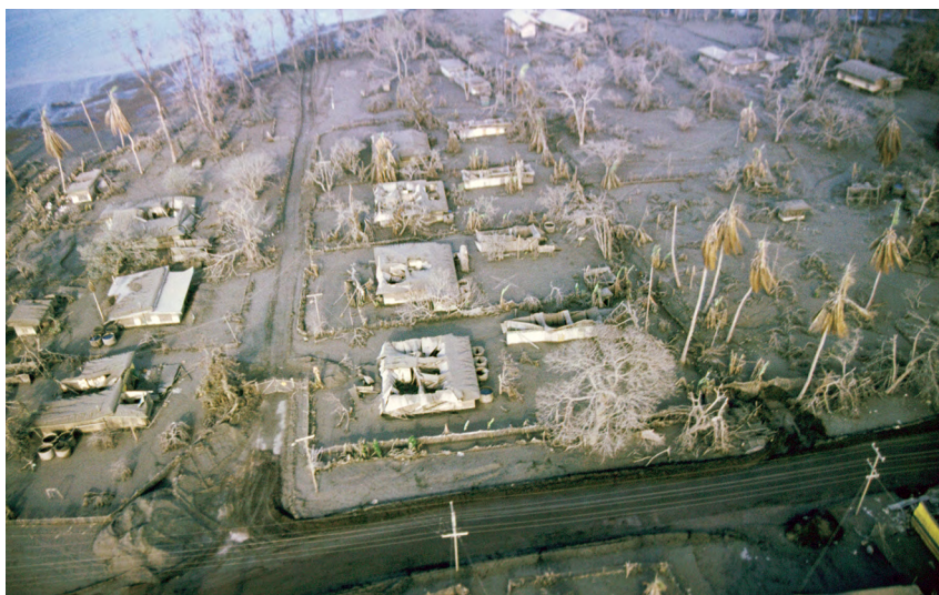
Figure 8.8. Close-up aerial view of roof and tree damage in Rabaul town.
