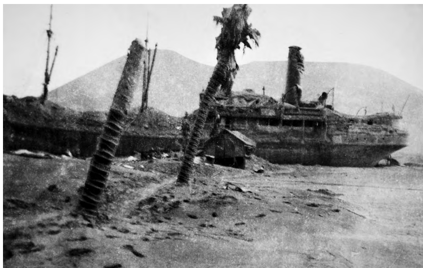
Figure 3.56. The Durour on the slipway in front of the new Vulcan cone.
