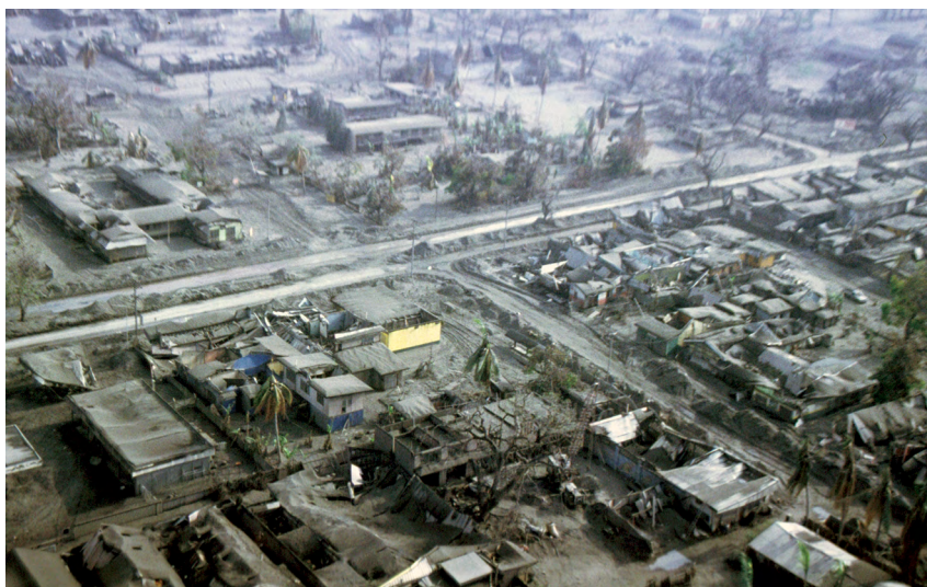
Figure 8.7. Aerial view of ash damage in northern part of Rabaul town.
