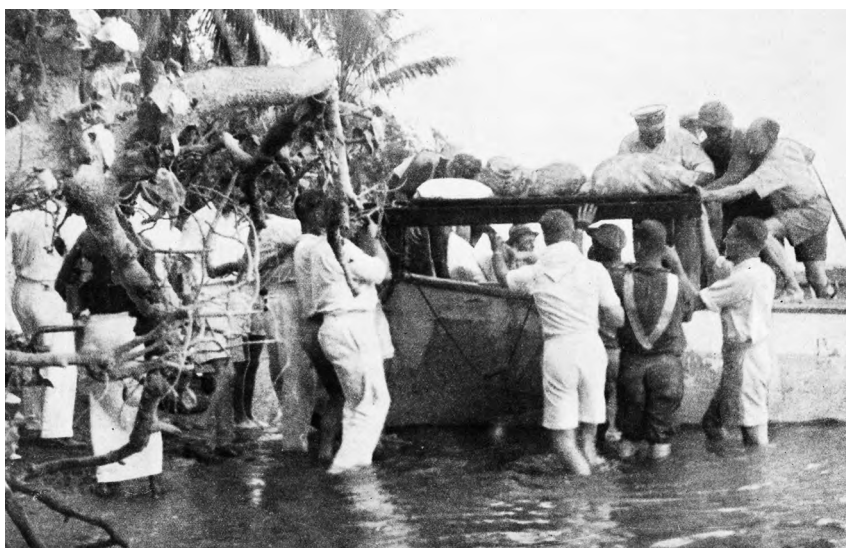
Figure 3.29. Launch being unloaded at Kokopo beach.
