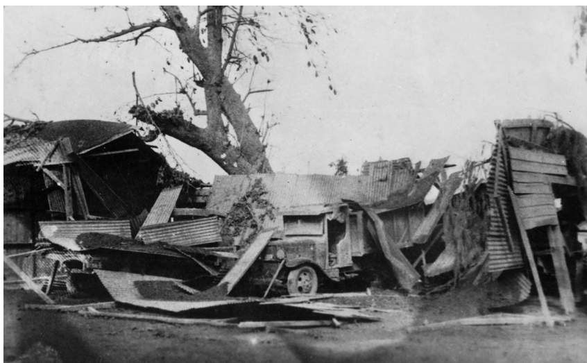
Figure 3.49. Roof collapse caused by ash loading.
