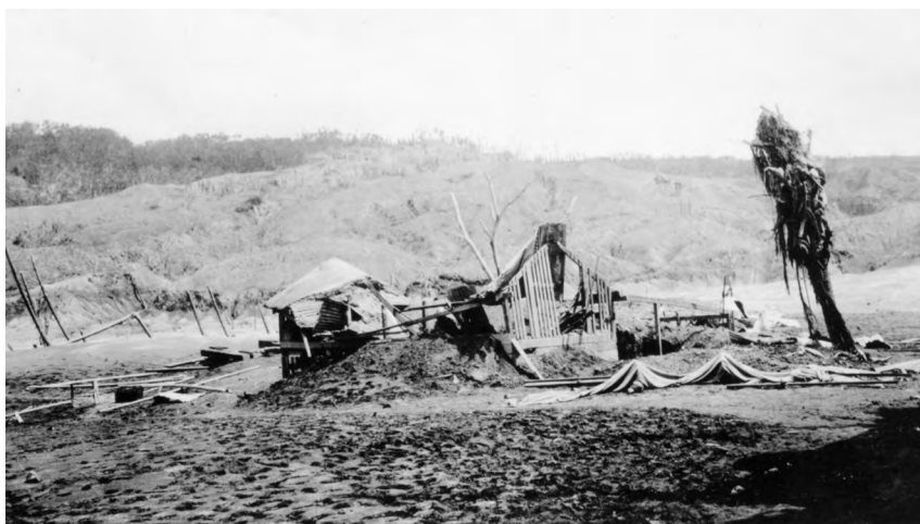
Figure 3.58. House collapse caused by volcanic ash from Vulcan.
