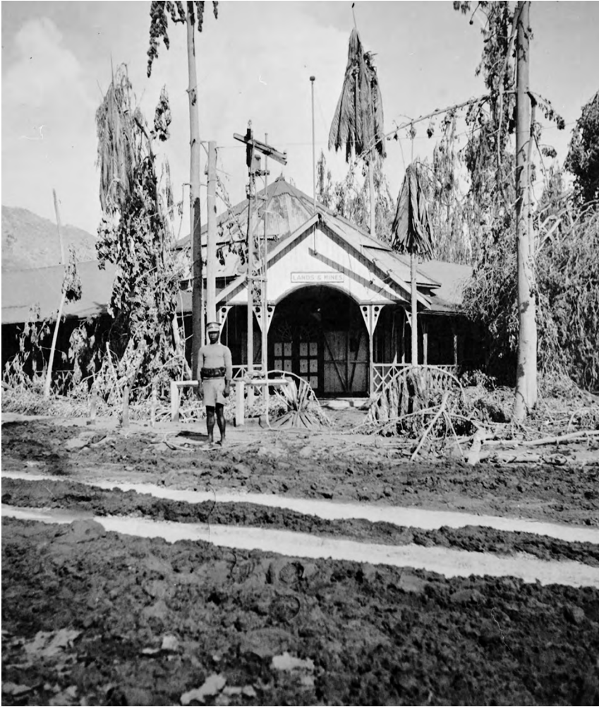
Figure 3.46. Department of Lands building and palm damage.
