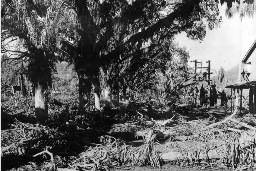
Figure 3.43. Malaguna Road damage.
