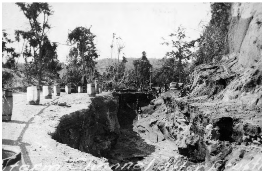
Figure 3.63. Erosion on Namanula Hill Road.
