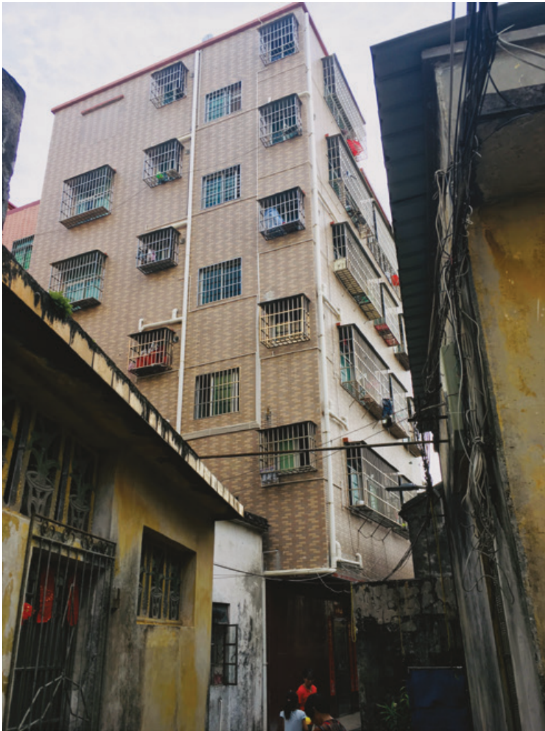
Figure 11.5.1 Small property rights housing on village residential plot in Zhuhai, Guangdong province. © Cinzia Losavio.
