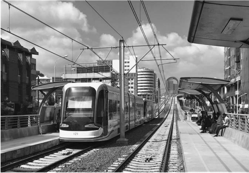
Figure 5.6 Addis Ababa LRT after construction
