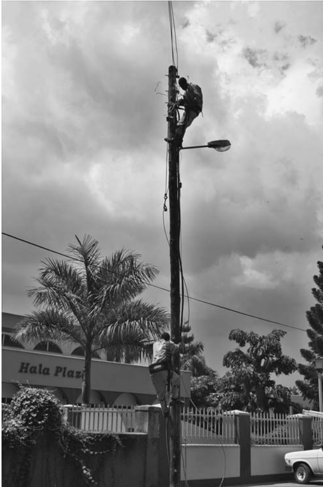
Figure 5.1 Infrastructural repair in Kampala Photograph © Tom Goodfellow.
