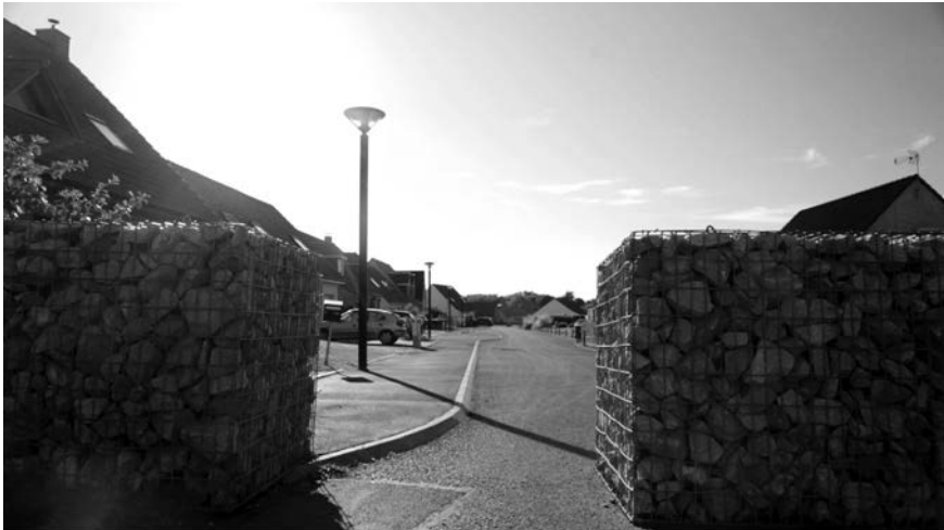
Figure 3.2 The gabion wall blocking vehicle access to Konin I district in Hénin-Beaumont.
