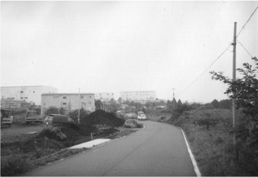
Figure 3.1 Satyam buildings in Kamikuishiki. Photograph by Yoshikawa Yūsuke, 1996. Reproduced under CC-BY-SA-4.0.
