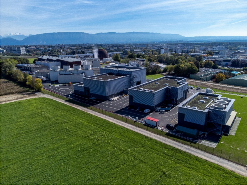
Fig. 19. Aerial view of the HL-LHC work site at Point 1.
