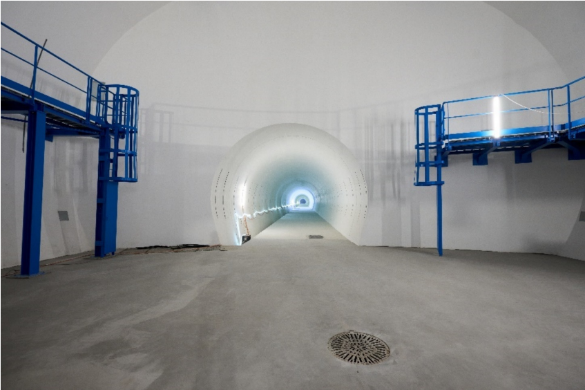
Fig. 20. HL-LHC underground cavern at Point 5.
