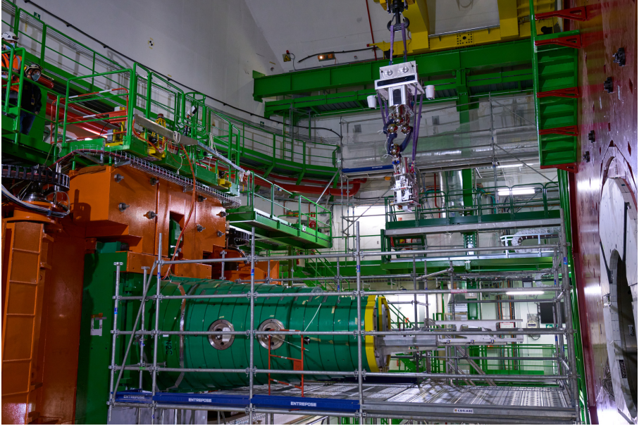
Fig. 7. The CERN CRANEbot is seen here carrying a VAX module (centre of the image) inside the CMS cavern, as part of an operation test conducted in early February 2021.
