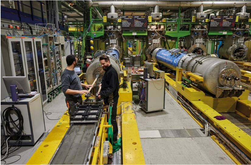
Fig. 7. Two first 11 T dipoles of the series production under test at the CERN testing infrastructure called SM18.
