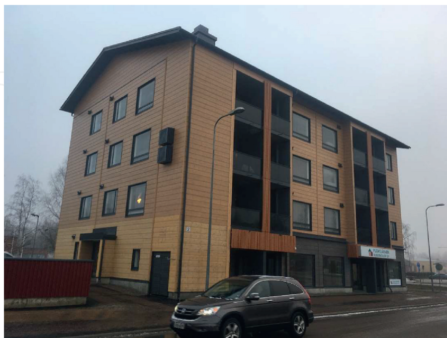
Figure 7. A four-story log apartment, Finland (photo by Hüseyin Emre Ilgın).
