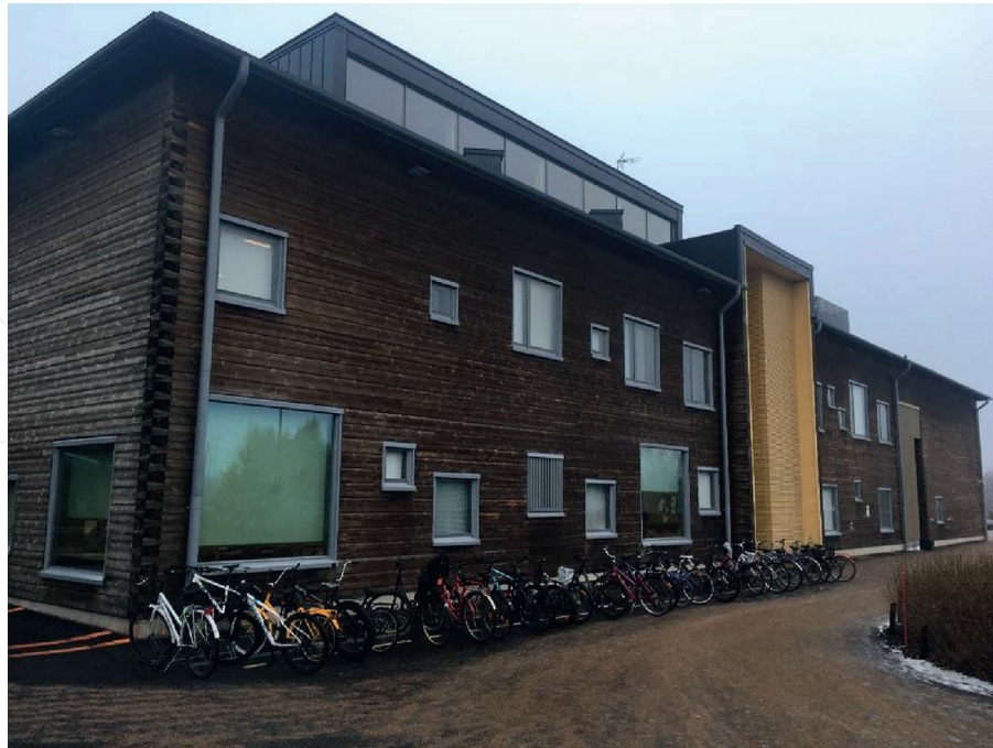
Figure 8. Pudasjärvi log school campus, Finland (photo by Hüseyin Emre Ilgım).
