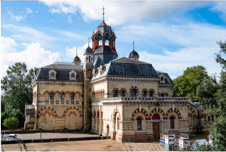
Figure 4.4 Edmund Cooper and Charles Driver, Abbey Mills Pumping Station, East London, 1865–8. © Simon from London. Wikidata, CC BY 2.0. Available at https://www.wikidata.org/wiki/Q4664040#/media/File:Abbey_Mills_Pumping_Station_(51551458944).jpg
