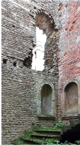
Figure 1.23: Kirby Hall, Northamptonshire. The south-east staircase tower, showing holes for supports for the collapsed landing on the first floor, south side, with the exit at the north-east corner through a doorway with a brick-lined arch.
