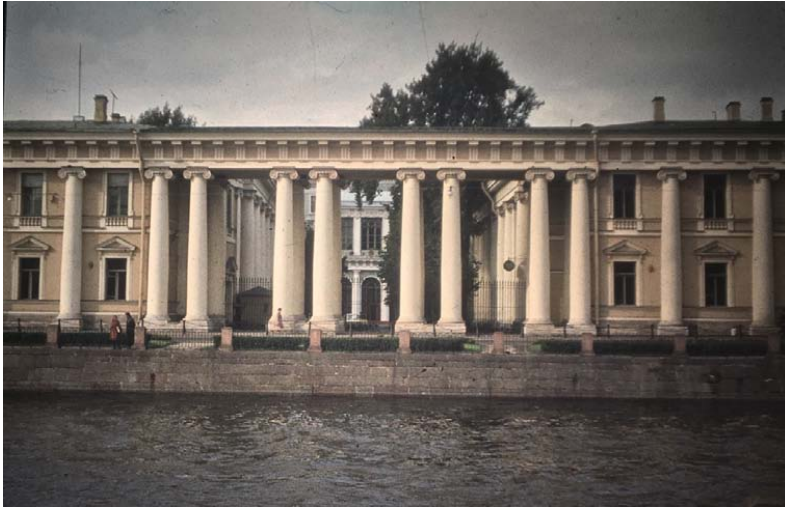
Figure 8.8: Giacomo Quarenghi, Anichkov Palace, St Petersburg. A range of shops along the Fontanka, commissioned 1803. The Doric frieze over Ionic columns is unconventional.
