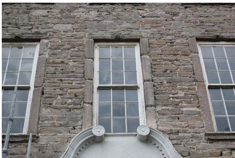
Figure 6.8: First-floor windows, Damer House.
