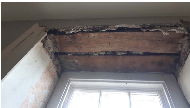
Figure 6.6: Timber lintels above window boxes, Damer House.
