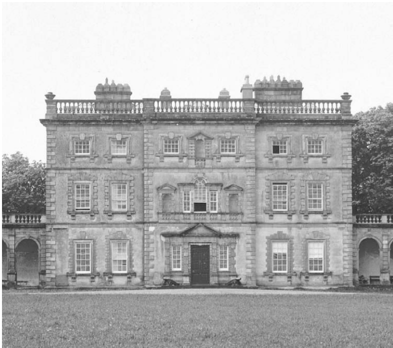
Figure 7.5: Entrance front of Florence Court, County Fermanagh, building from 1758. T. U. Sadleir and P. L. Dickinson. Georgian Mansions in Ireland , Plate LIII.
