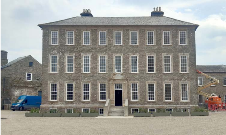
Figure 6.21: North façade, Damer House, following completion of repair work in April 2023.
