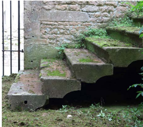
Figure 1.20: Kirby Hall, Northamptonshire. The first flight of the south-east staircase. Detail.
