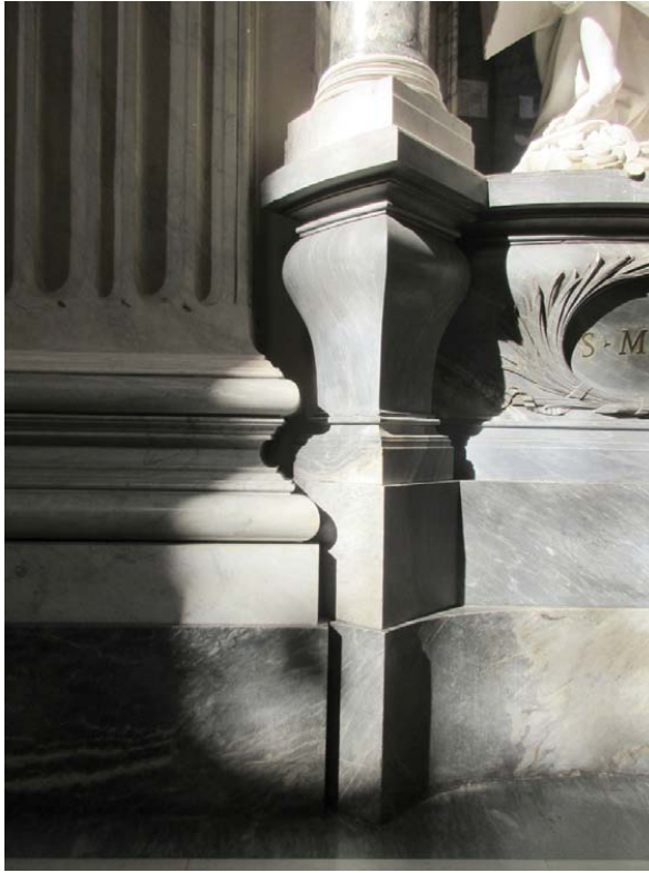
Figure 8.2: Francesco Borromini, San Giovanni in Laterano, Rome, 1646–9, bases in the nave.
