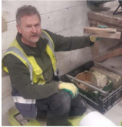
Figure 6.9: Master mason Gunther Wolters displays construction wedges used to support a timber lintel from the first-floor windows. Damer House.
