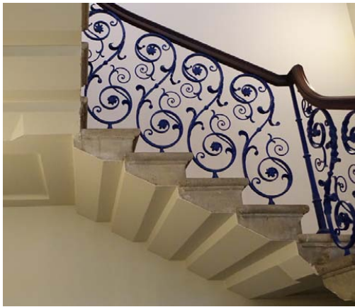
Figure 1.8b: The South Stair at the Queen's House. Central flight and half-landings, showing riser rebates and chamfered soffits.
