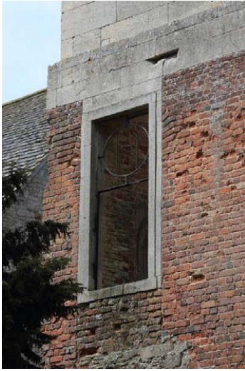
Figure 1.19a: Kirby Hall, Northamptonshire. Window in the south-east staircase tower.
