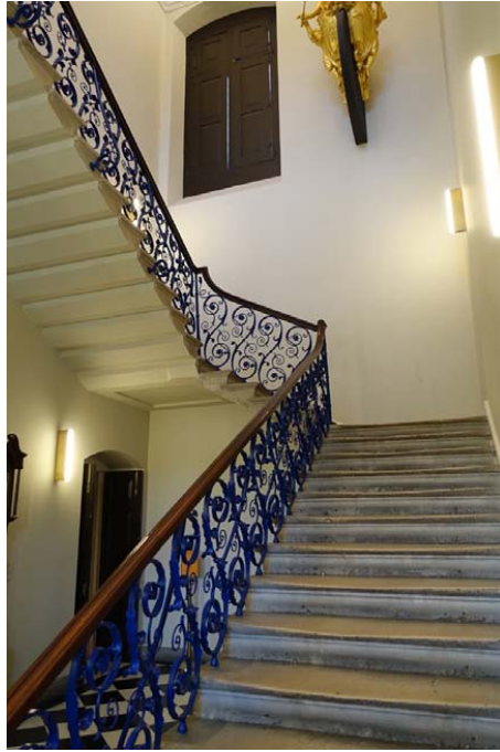
Figure 1.7: The South Stair at the Queen's House. Balustrade, circa 1760, installed in 1936.
