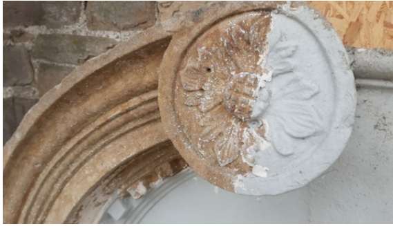
Figure 6.15: Sample cleaning portion of doorcase with decorated floral scroll, Damer House. The scrolls are enriched with cyma recta consoles, forming a deep reveal enriched with dentils. The frieze is supported on fluted pilasters with lively Corinthian capitals and plain bases. A cyma recta curve is also a feature of the window surrounds.
