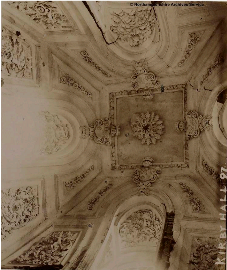
Figure 1.17: Kirby Hall, Northamptonshire. The plaster ceiling of the south-east staircase tower before its collapse.
