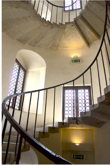
Figure 1.3: Palladio's oval stair at the Convento della Carità, Venice (now the Gallerie dell'Accademia), early 1560s. Windows and landing at second-floor level.
