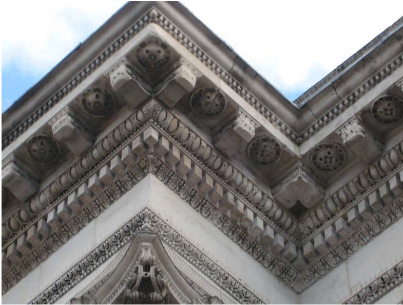
Figure 8.4: Thomas Cooley, Royal Exchange, Dublin (now the City Hall), 1769–79, detail of cornice with merged modillions.
