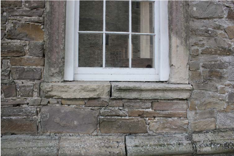
Figure 6.7: Window sill, Damer House.
