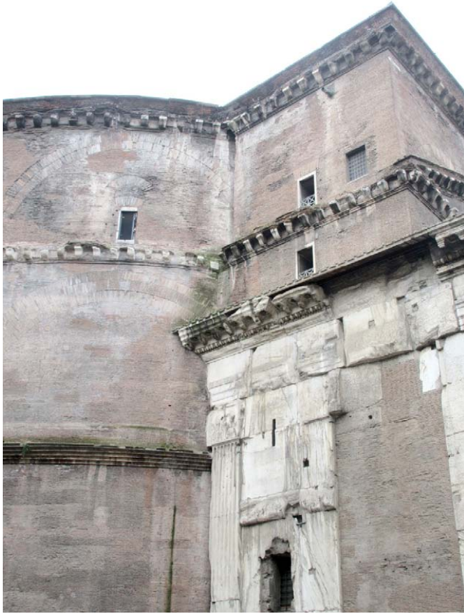
Figure 8.7: Pantheon, Rome, early second century, the discontinuity between portico and body of the temple is believed to be due to a change of intention during erection.
