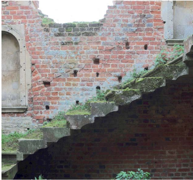
Figure 1.21: Kirby Hall, Northamptonshire. The second flight of the south-east staircase, showing holes made for panelling and the line of a wooden balustrade.
