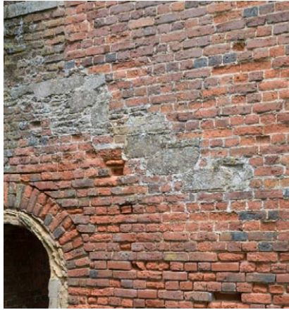
Figure 1.22: Kirby Hall, Northamptonshire. The south wall of the south-east staircase tower from outside, showing the treads of the staircase flush with the wall.
