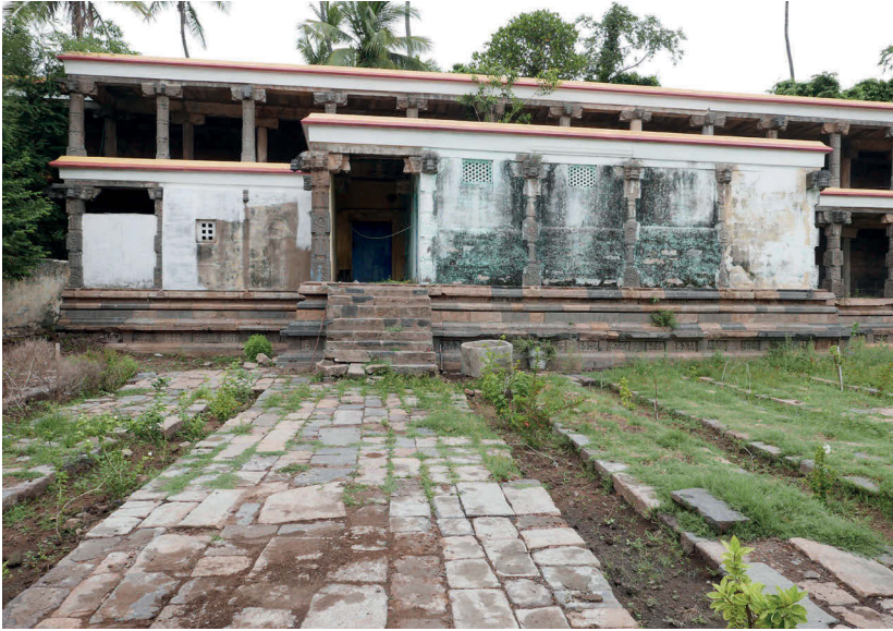
Fig. 5a: View from the east: from the foreground, the garden, the five-intercolumniated long library's pavilion with the new staircase and (to the left and rear in the gallery) the extension of the library.
