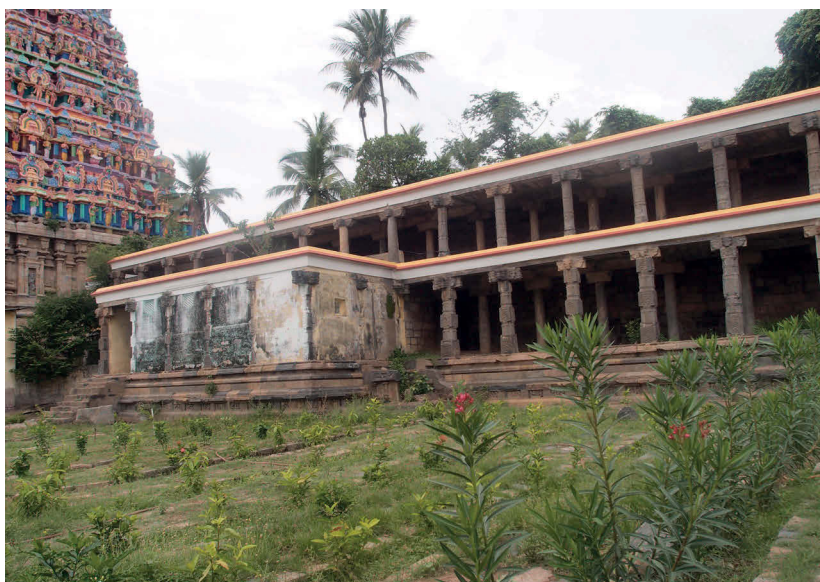
Fig. 4b: View from the north-east: the gallery where the library is located and adjoined with its projecting pavilion (old staircase on the right (north) side) and the garden around.
