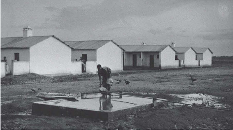
4 Workers' neighborhoods in Caingagi, Lunda, 1960.
