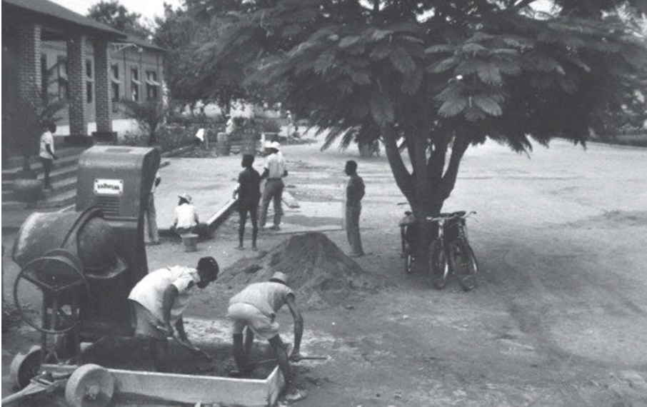
6 Construction works at Dundo's hospital, 1961.
