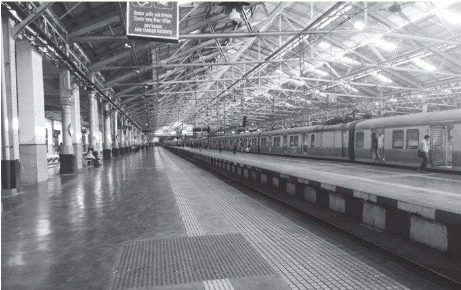
2 View of the station shed today; original columns visible.
