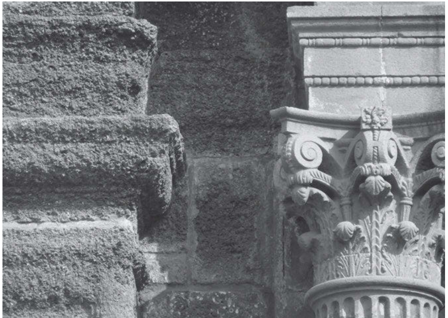
5 Detail of the condition of the laterite stone (left) compared with the granite stone (right) (2018).
