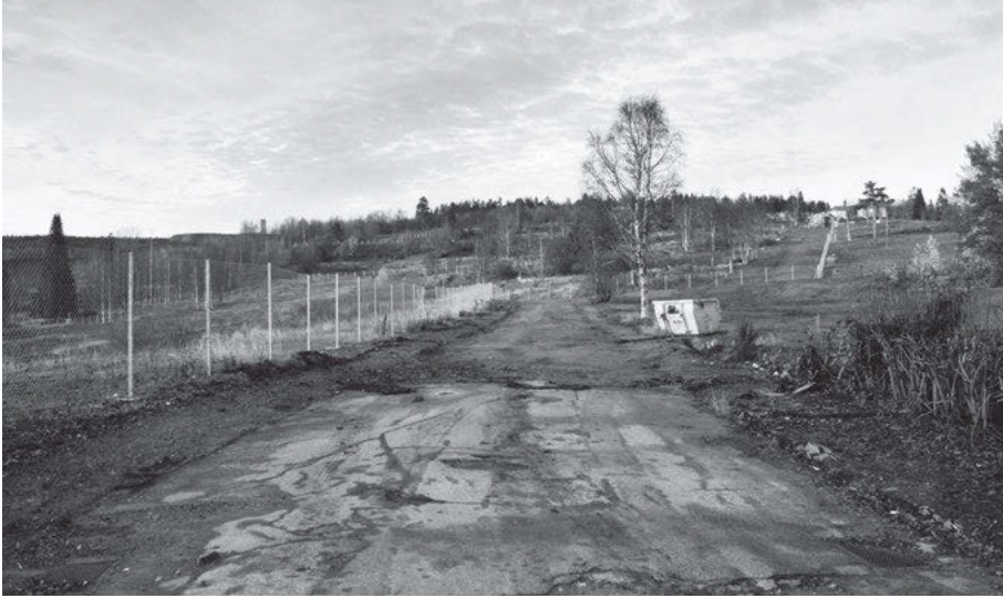
4 Malmberget Östra (Eastern Malmberget) with around 75 % of the houses already demolished, 2021.
