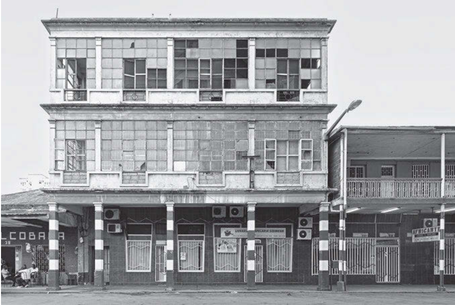
5 Building in old downtown area, Rua da Mesquita, Maputo, 2011.
