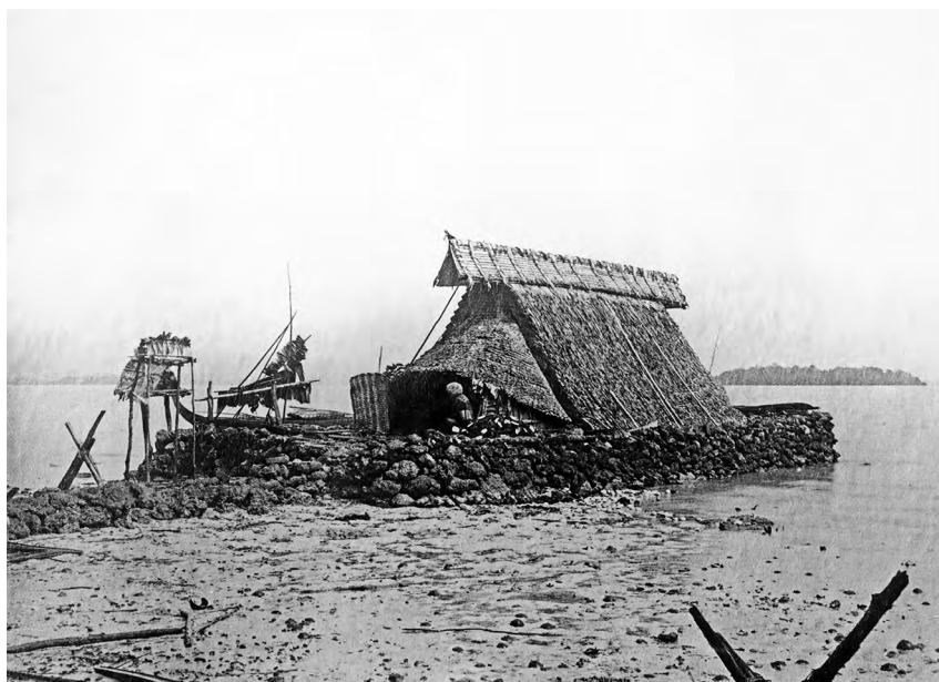
Figure 4.6: House on rock foundation in the tidal zone of Babata, Tusu Marovo, early 1890s
