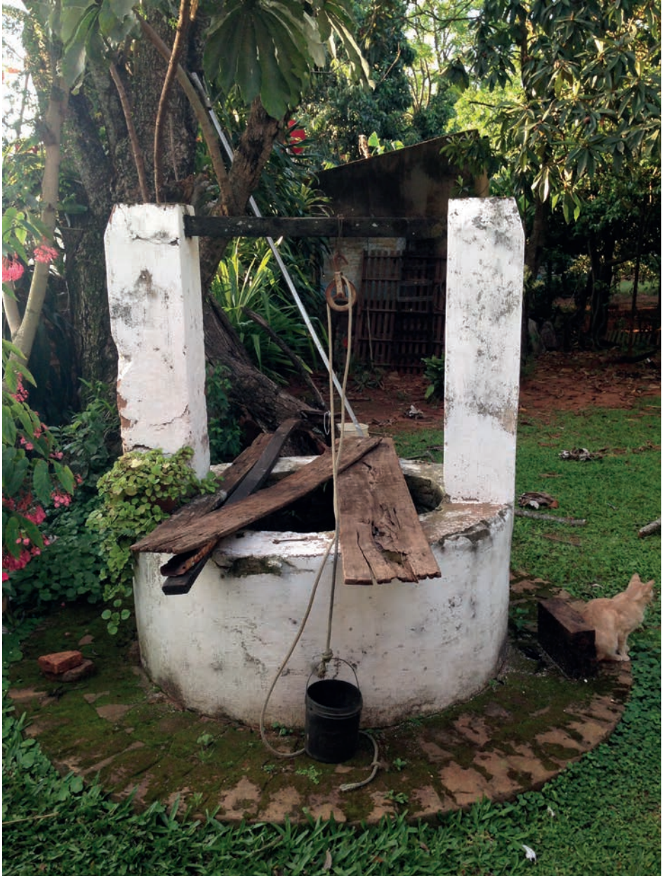
In order to obtain fresh water, they have built a 12-meter-deep well—also using manual tools only.
