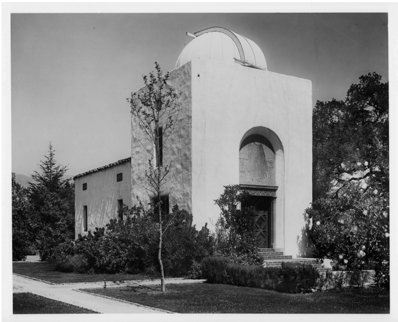
Figure 6.9 Hale Solar Observatory in Pasadena, California (1924, photographed 1931), architect Johnson, Kaufman & Coate. Photo credit: Observatories of the Carnegie Institution for Science Collection at the Huntington Library, San Marino, California.
