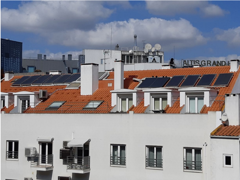
Figure 7.10 Neatly integrated limited solar PV atop middle class Lisbon buildings. © The author
