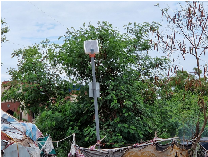
Figure 7.2 Solar PV integrated in Jaipur's street lighting above a shanty. © The author
