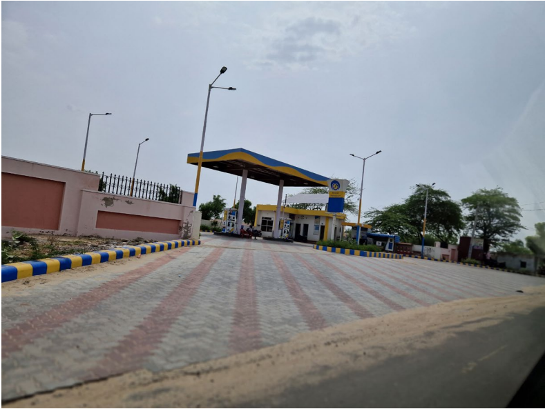
Figure 7.3 Solar PV is ubiquitous at fuelpumps in Jaipur. © The author
