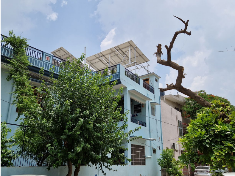
Figure 7.1 Solar PV atop middle class housing in a Jaipur suburb. © The author
