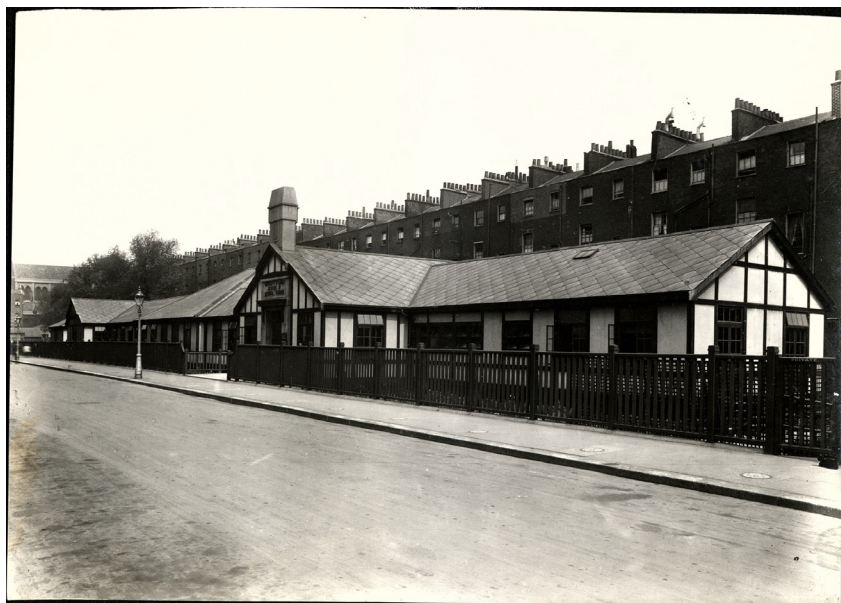
Figure 1.2 The temporary building for the IHR on Malet St, London, 1926; creator unknown. Institute of Historical Research, Wohl Library: IHR 10/1/2. Reproduced by kind permission of the Institute of Historical Research's Wohl Library.
