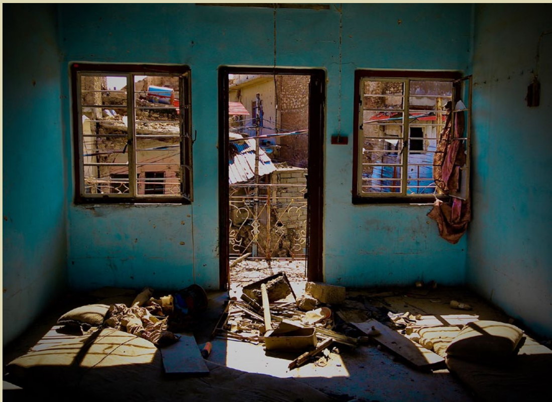
The sleeping area in a residential building formerly occupied by Islamic State 2019
