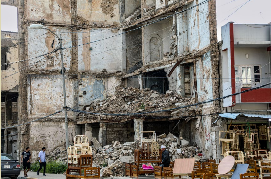
Completely destroyed building about a block away from the fish market 2023
