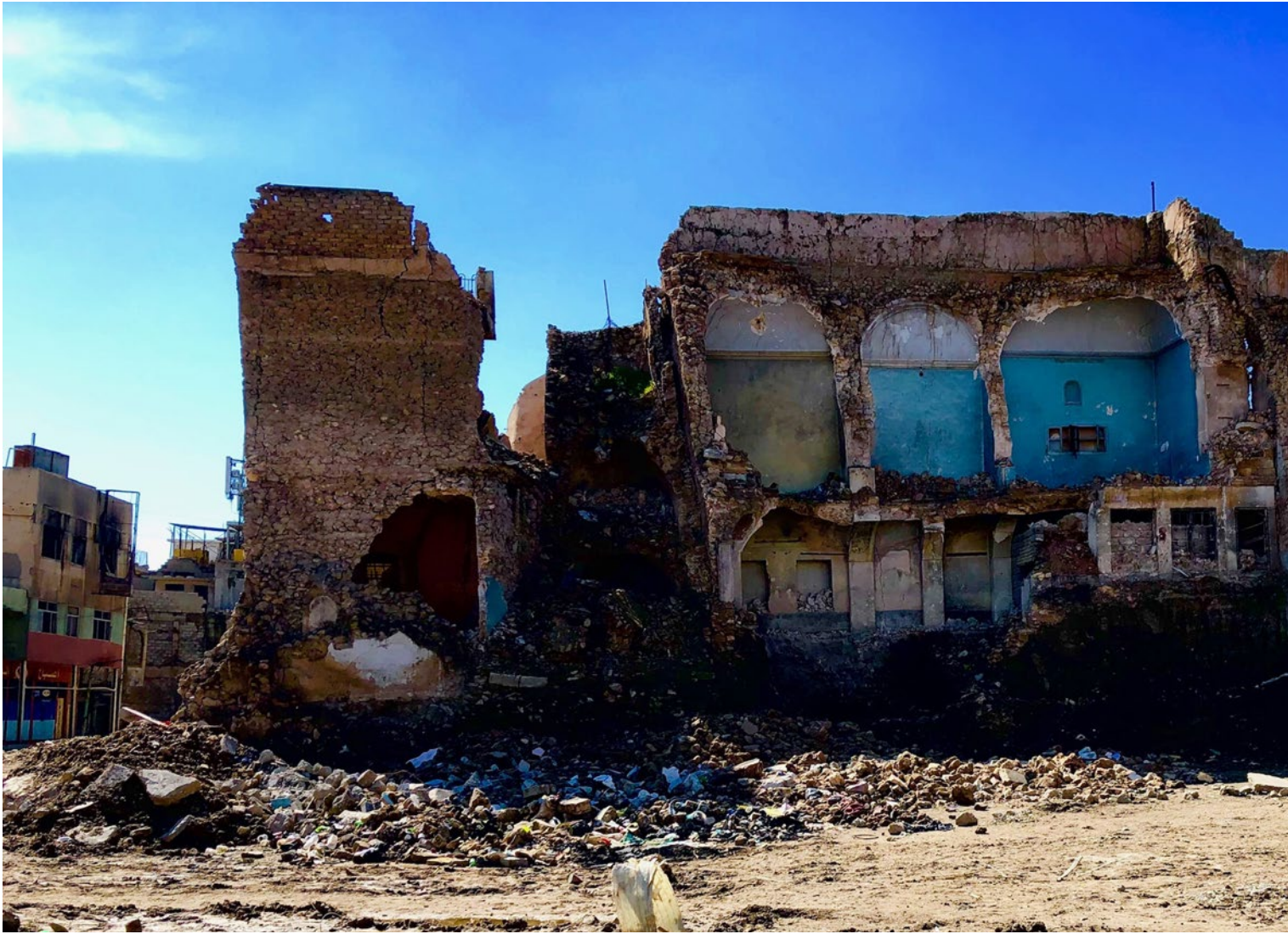
A destroyed residence 2019
