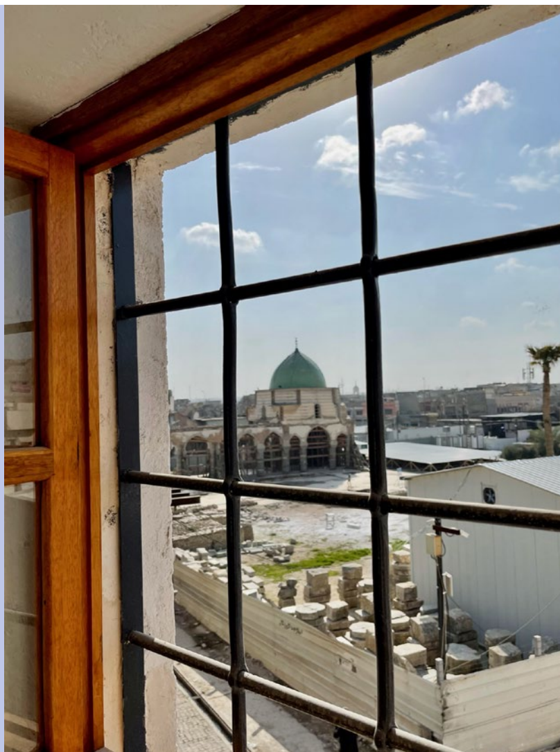
Renovated home next to the reconstruction site of the al-Nuri Mosque 2022
