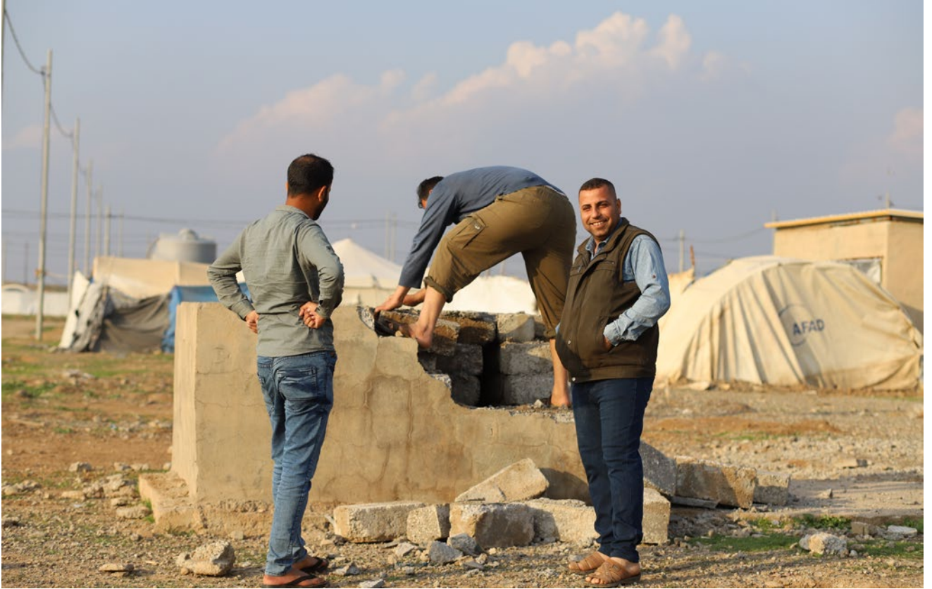
Demolition of a structure 2022
