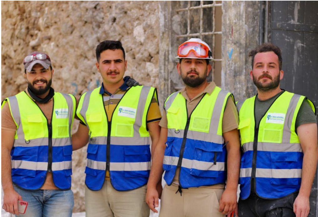
Construction workers from the Mosul Heritage Group renovating the area around the al-Nuri Mosque 2023
