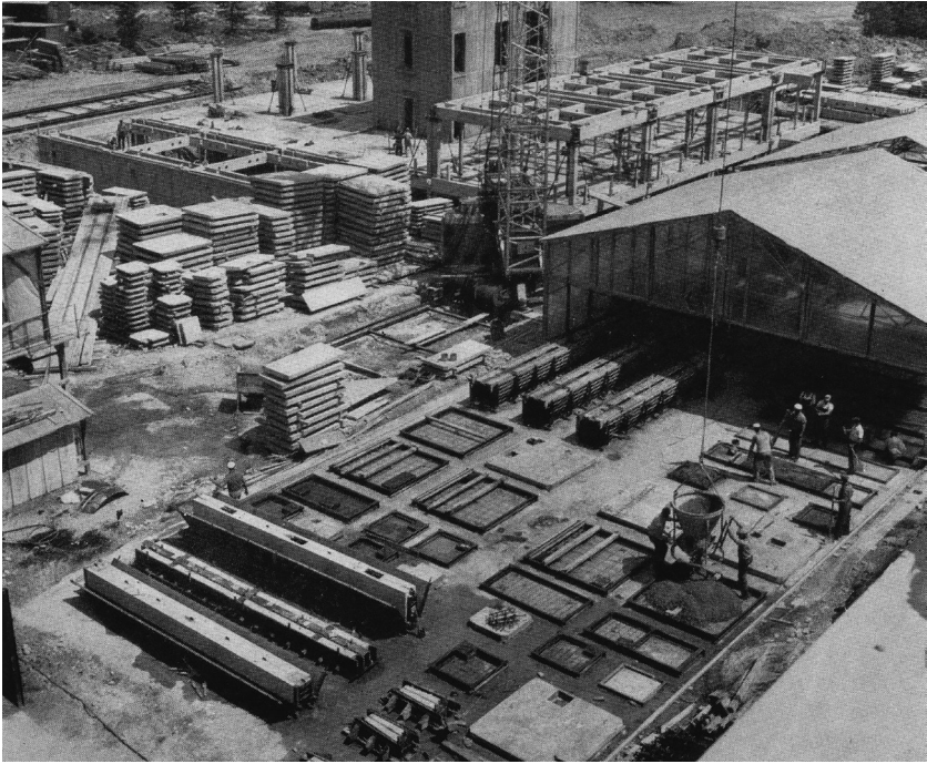
Fig. 11.3. Field factory for producing system components on the construction site of the University of Marburg. Hochtief Nachrichten , December 1964.
