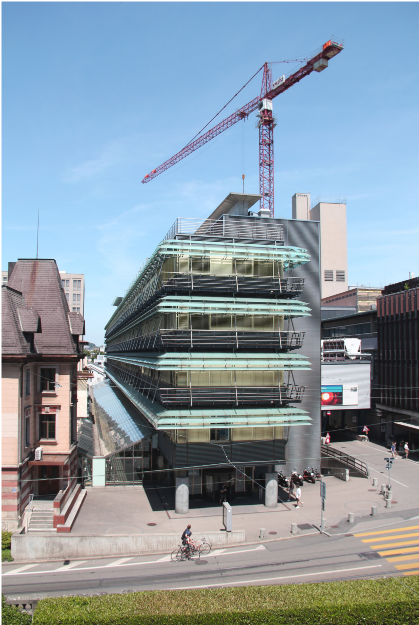
Fig. 11.4. The filigree high-tech facade of the institute building on Clausiusstrasse “CLA” of ETH Zurich is constructed from special metallic components. Matthias Brenner, ETH Zurich.
