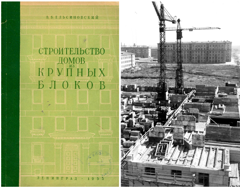
Fig. 6.1. Large block construction: the Elsinovsky's manual (left) and a view of Kvartal no. 21 in construction (right) in Leningrad [Elsinovsky, 1955]. Source: Vladimir Elsinovsky. Construction of Houses from Large Blocks: Design, Production and Installation (Строительство домов из крупных блоков. Конструкции, производство и монтаж). Moscow, Leningrad: Gosudarstvennoye izdatel'stvo Literatury, Stroitel'stva i Arkhitektury, 1953, Cover and page 15.
