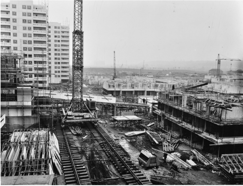
Fig. 7.3. Thamesmead: Harrow Manorway under construction, 1969. London Picture Archive, London Metropolitan Archives, LCC Photograph Library.
