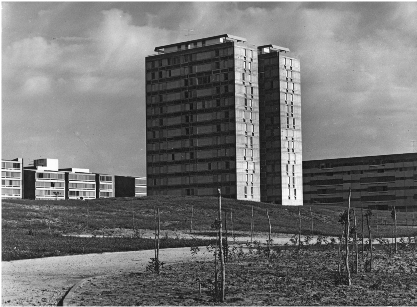
Fig. 5.2. Yisrael Lotan, Erich Bauman and Werner Joseph Wittkower Kiron Estate, Havatselet Tower, Kiryat Ono, 1962-1965. Source: Kiryat Ono Municipal Archive, photo by Komriner, 1965. https://www.pikiwiki.org.il/gallery/?s=%D7%A7%D7%99%D7%A8%D7%90%D7%95%D7%9F&method=exact&topic=8&page=2 . Accessed 2/4/2023.
