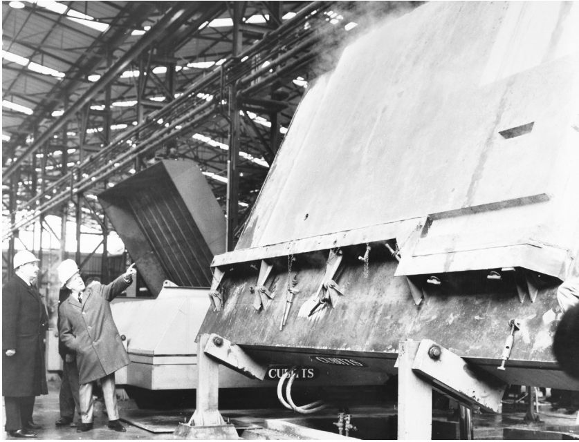
Fig. 7.2. Thamesmead Factory: Mr. Plummer looking at concrete wall of a house, just coming out steaming hot, 1968. London Picture Archive, London Metropolitan Archives, LCC Photograph Library.
