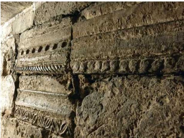
Figure 5.5: Decorated Roman stone blocks in the 7th-century crypt at Hexham Abbey, re-used from Roman buildings at Corbridge.
