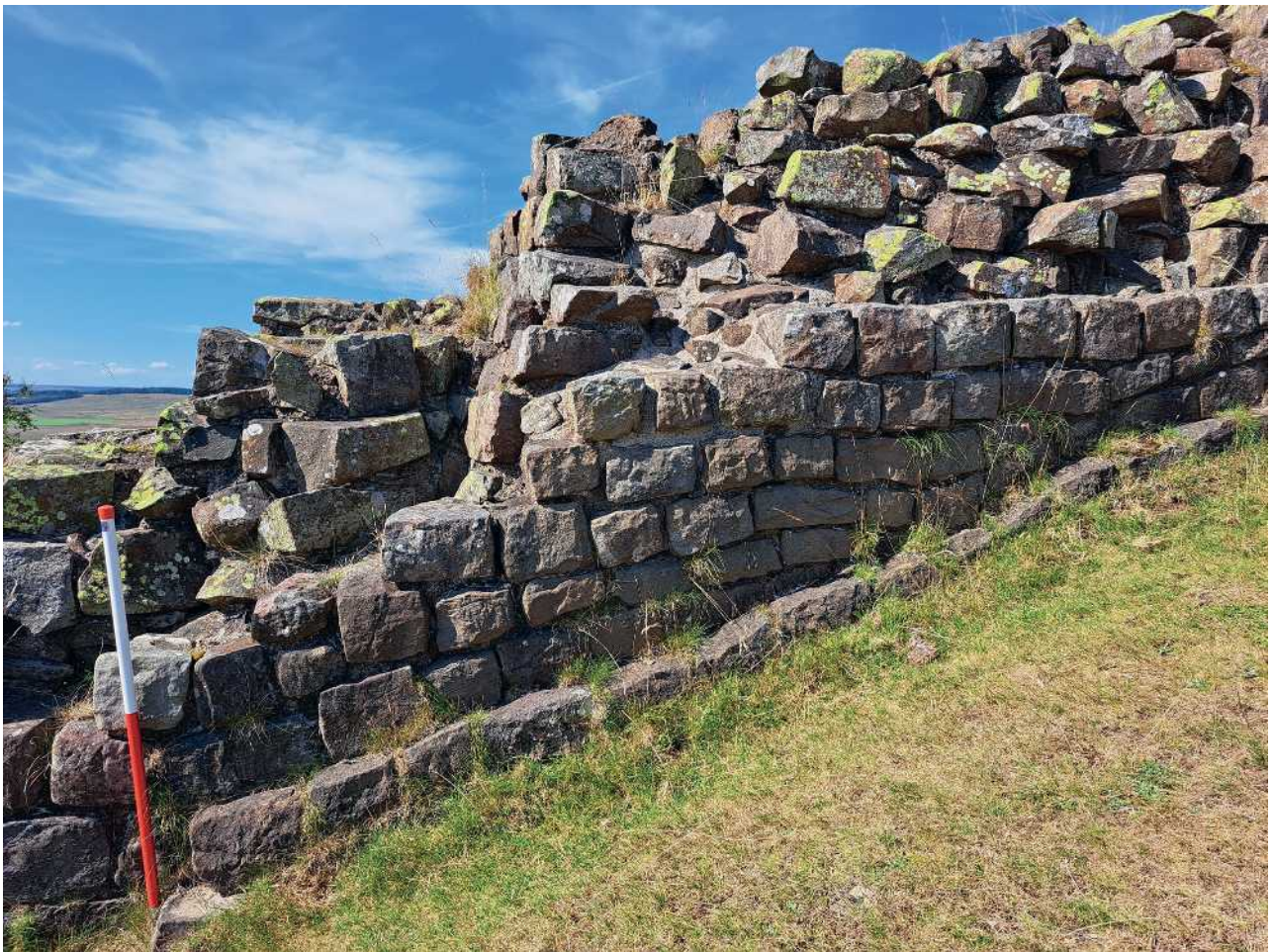
Figure 3.12: The south face of the curtain at Walltown Crags, where it runs down a slope to the west. Note how the foundation stones generally parallel the slope of the ground, while the stone courses above mix sloped coursing and even coursing, rather than stepped coursing that cuts into the slope. The scale bar is 1 m.
