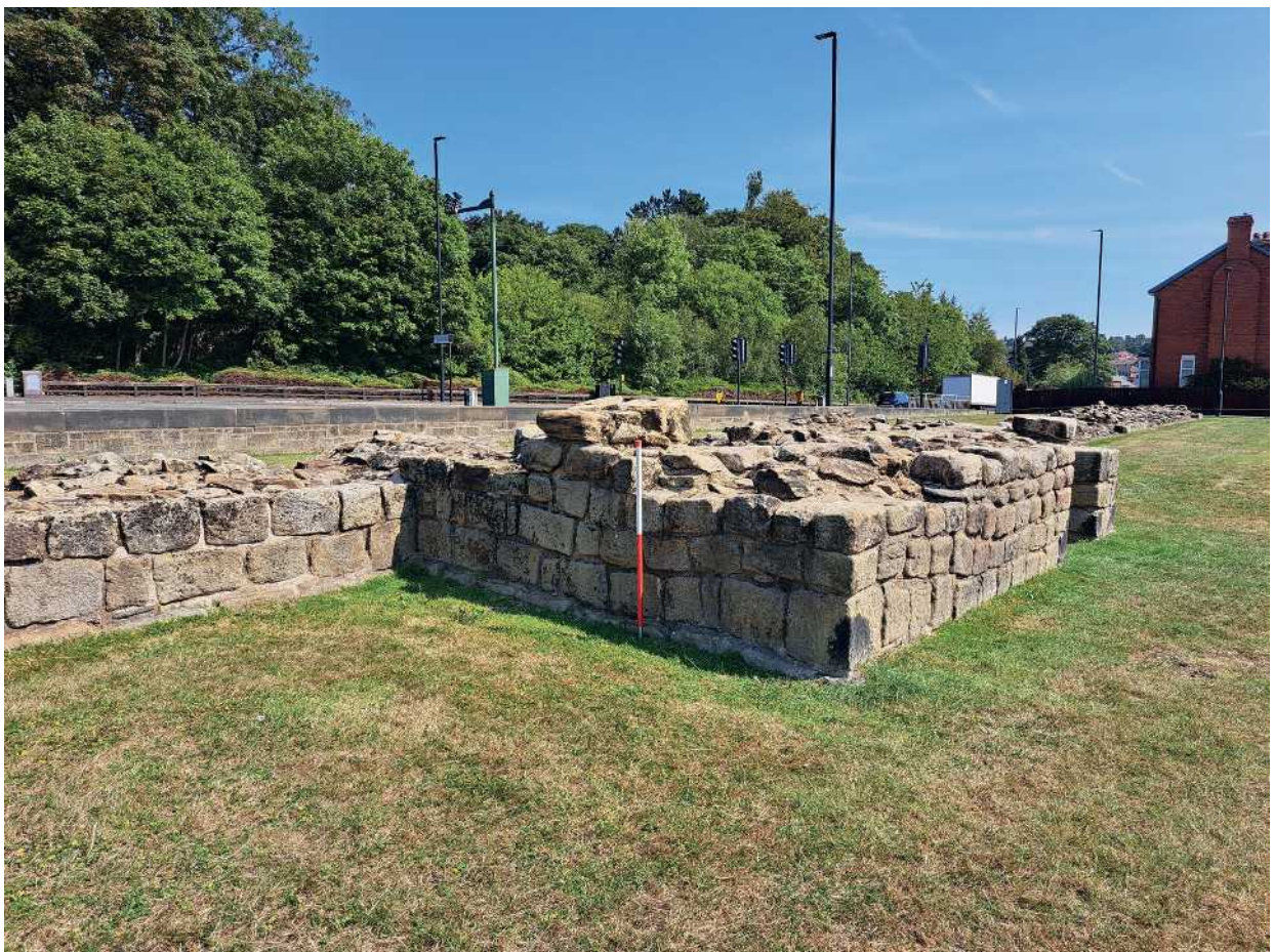
Figure 3.15: Denton turret 7b, as viewed from the southwest. Note how the southern and western external faces have been consolidated, fixing the slump of coursing. The larger stones visible in the southwest and southeast corners and the south face of the curtain are in situ Hadrianic fabric, while the smaller stones that make up the south and west turret faces are rebuilt. The scale bar is 1 m.
