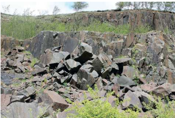
Figure 4.28: Angular rubble as a result of blasting at Cawfields Quarry.
