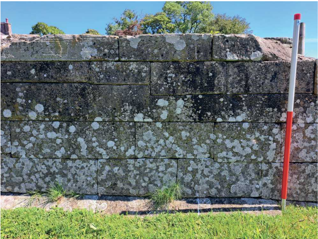
Figure 3.7: Ashlar used at the east gate of Birdoswald fort. Note the high-quality finish to the faces, beds, and joints of each stone, ensuring a tight fit. Scale bar is 1 m.
