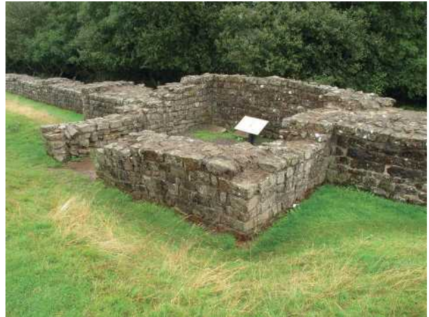
Figure 1.10: Turret 48b, east of Willowford Farm, looking into the low surviving courses of the structure from the southeast.
