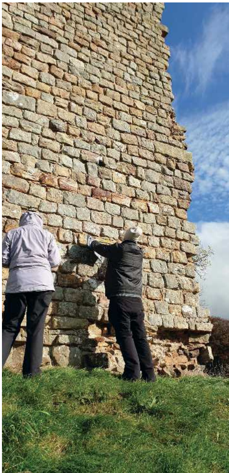
Figure 1.2: WallCAP volunteers recording stone fabric at Thirlwall Castle, taking note of morphological and metric aspects of the stone for its use as a building material, and geological attributes of the stone that help to identify its origins and sourcing.
