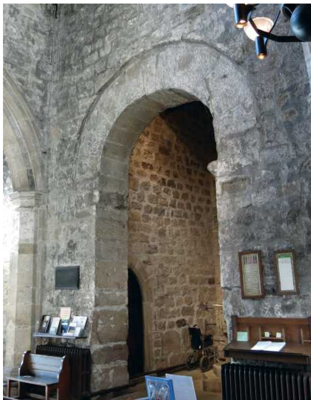
Figure 6.1: A re-used Roman arch, complete with piers, springers, and voussoirs, erected between the nave and the tower at St Andrew's, Corbridge, probably built in the 9th–10th century.
