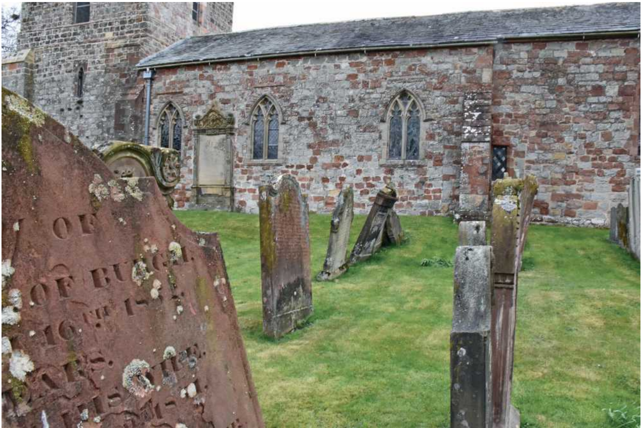
Figure 2.29: Possible re-used Wall stones of St Bees sandstone at St Michael's Church, Burgh-by-Sands. Gravestones also made of St Bees sandstone.
