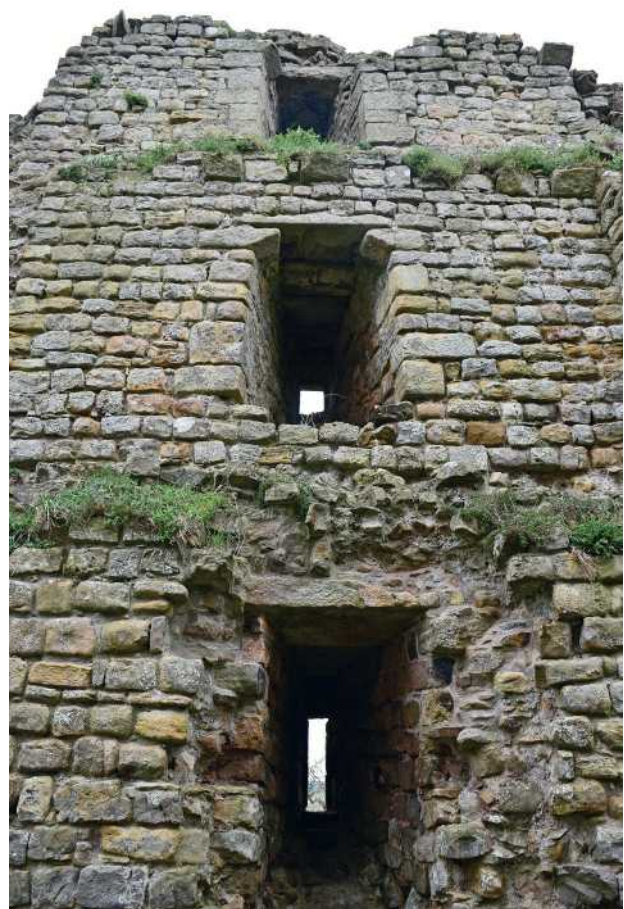
Figure 5.7: The internal face of the south wall of Thirlwall Castle, highlighting the consistent fabric in different sandstones.
