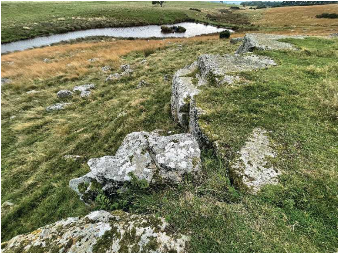
Figure 4.25: The stepped pattern of block removal partially visible under overgrowth at Fallowfield Fell, Northumberland.
