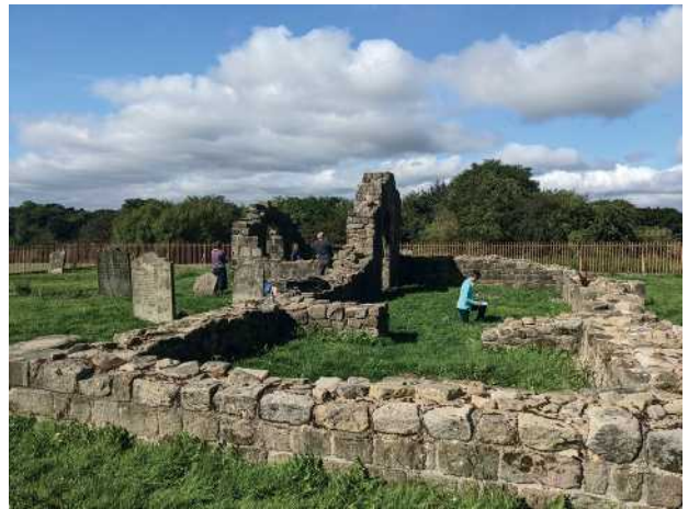
Figure 5.10: The consolidated ruins of Holy Cross Church, Wallsend, located north of the line of Hadrian's Wall. Though largely robbed, some of the remaining stone is re-used Roman fabric.
