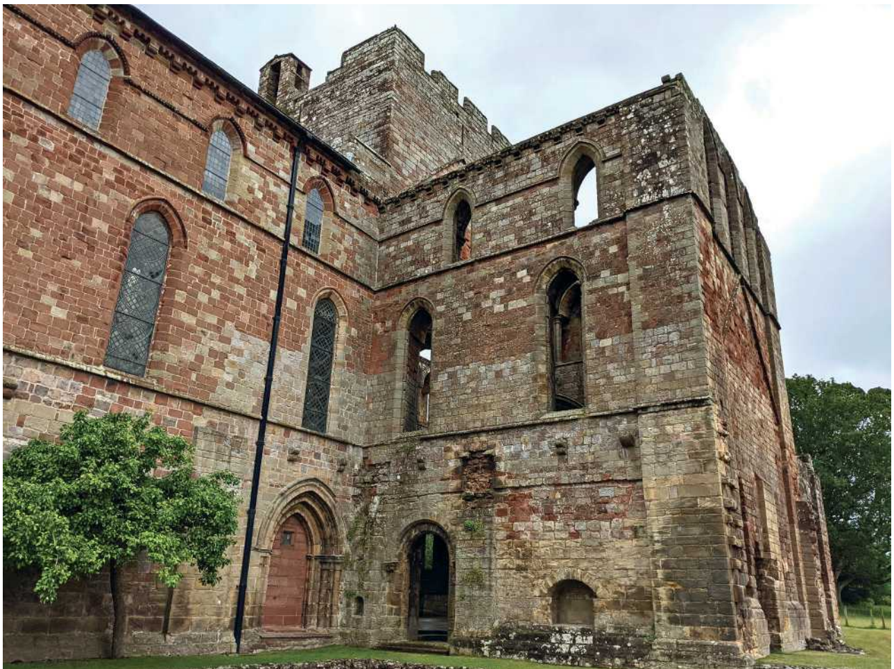
Figure 5.11: The south wall of the nave and west wall of the transept at Lanercost Priory, which makes extensive use of red and white sandstones from Hadrian's Wall.
