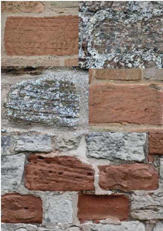
Figure 2.4: Examples of the range of colours and textures in Wall-stones from the St Bees Sandstone Formation in the Triassic strata.
