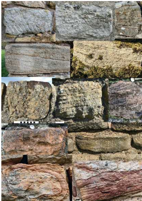
Figure 2.2: Examples of the range of colours and textures in Wall-stones from the Carboniferous strata.
