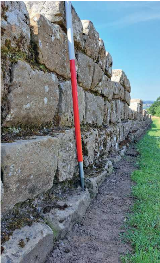
Figure 3.9: The north face of the curtain at Planetrees, with first course over the foundations providing a single-footing. Scale bar (red section) is 50 cm.
