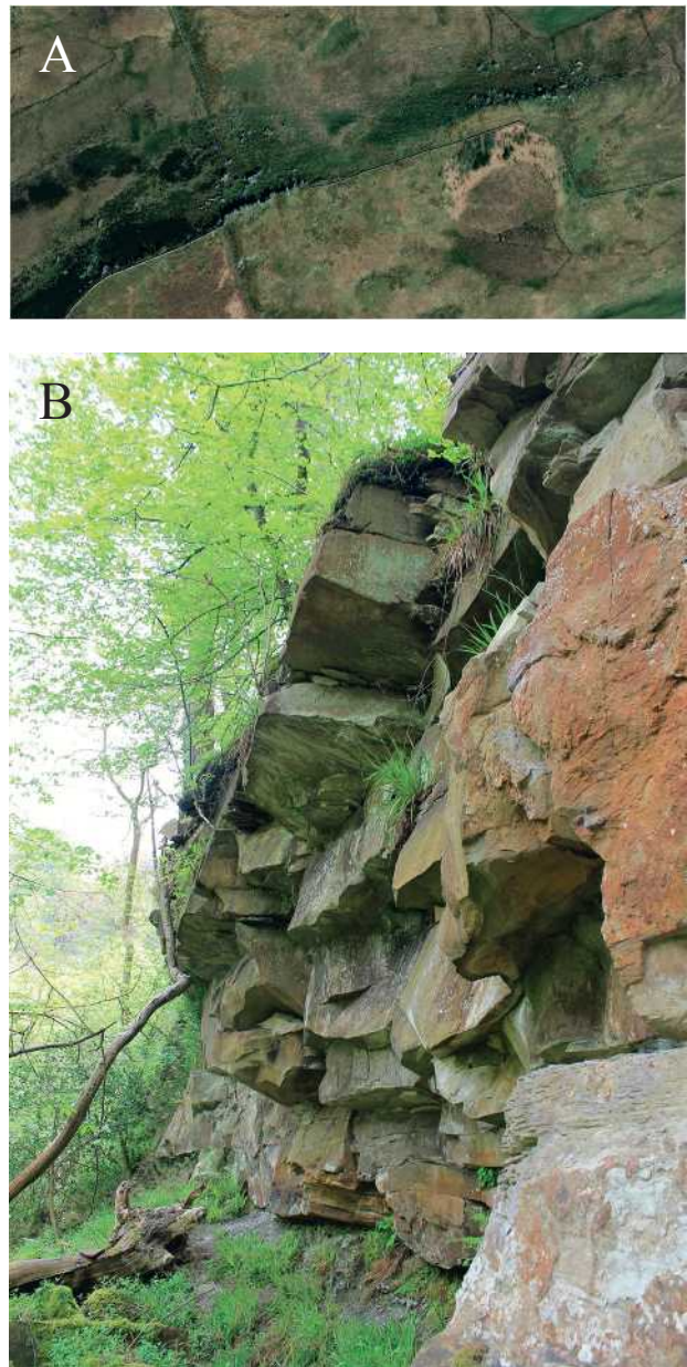
Figure 4.27: (A) Satellite imagery of the quarry face at Queen's Crag. © Apple Maps. (B) The overhanging rock on the quarry face at Comb Crag, Cumbria.
