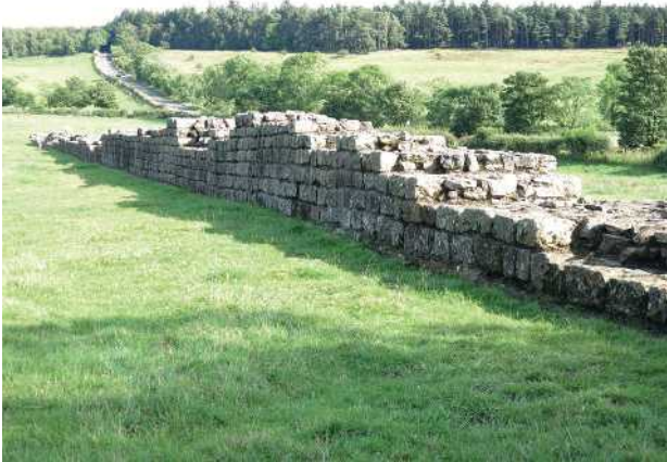
Figure 1.6: The gently rolling hills that flank the upland central sector of the Wall are visible at Black Carts, looking east from the north side of the curtain.
