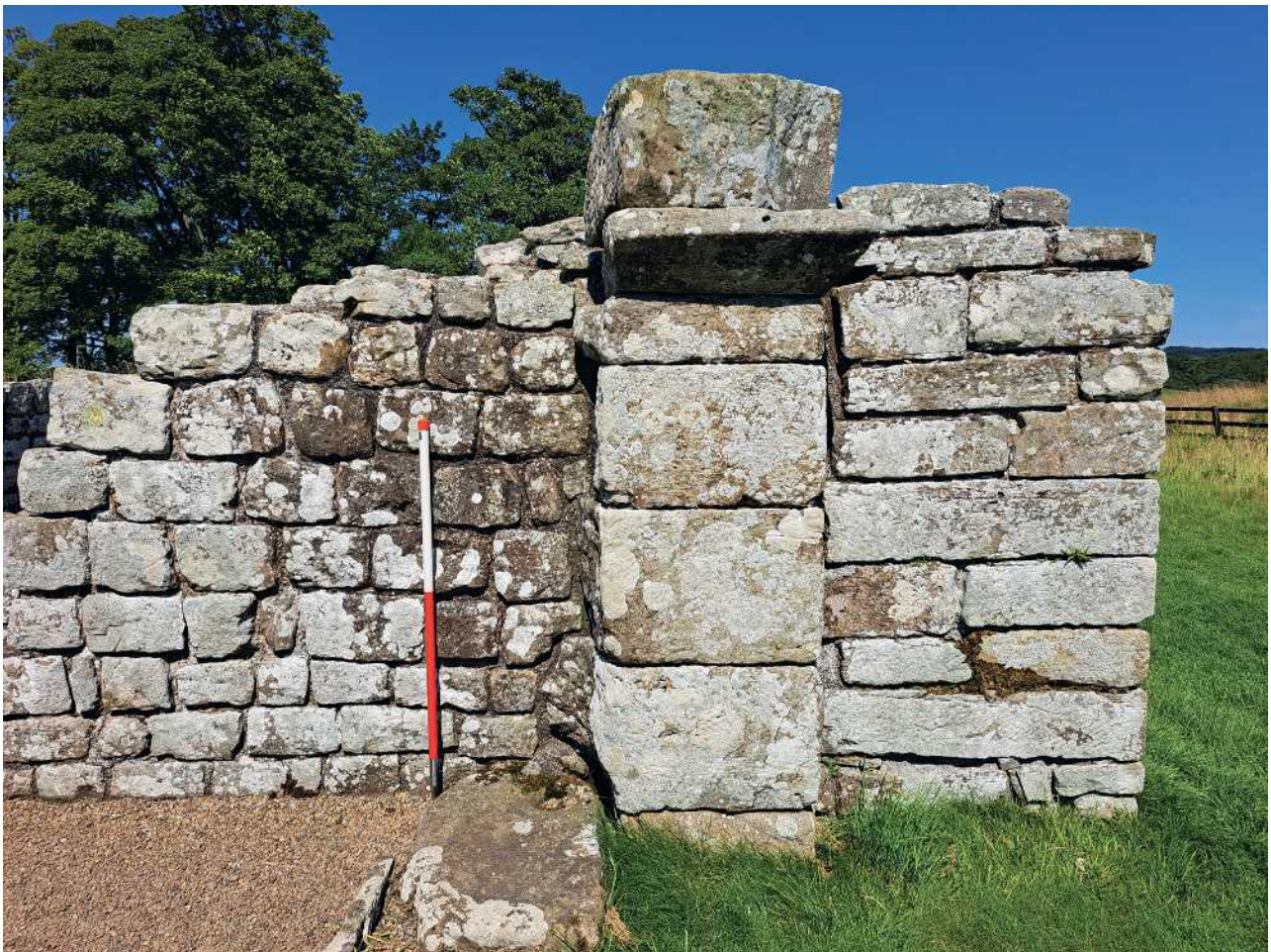
Figure 3.6: The north portal of the east gate at Birdoswald fort, showing the use of block-in-course construction for the outer fort walling and gate pier (right) while squared rubble is used for the internal gate walling (left). Scale bar is 1 m.
