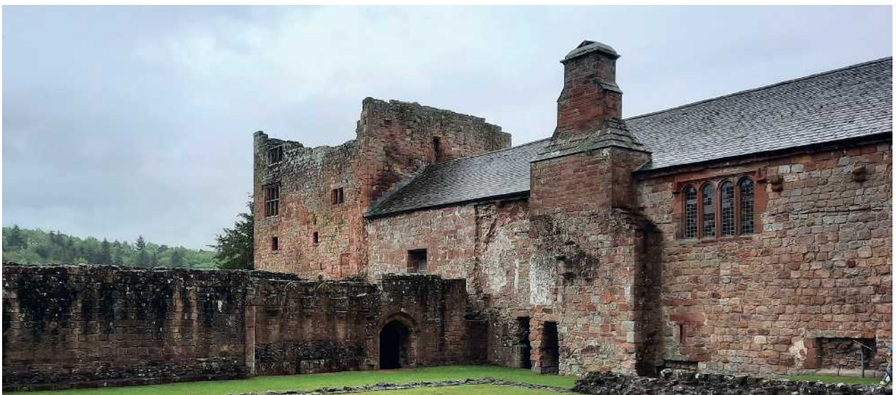
Figure 5.13: The west and south wings of the enclosed cloister of Lanercost, with the west wing and tower built substantially of red sandstone. White sandstones were used in the southern wing (crypt), though the colour is partially obscured by weathering.
