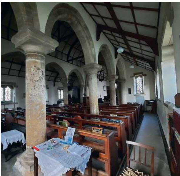
Figure 6.3: Roman columns used in the medieval south arcade of St Giles, Chollerton, probably dating to the 12th–13th centuries.
