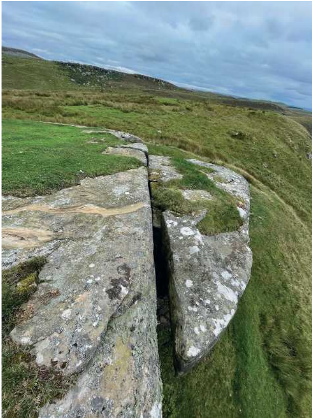
Figure 4.18: Linear cracks in weathered stone.
