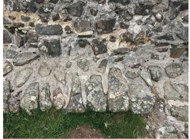
Figure 2.20: Triangular-shaped blocks of whinstone used in the foundations of the Wall at Sewingshields Crag.
