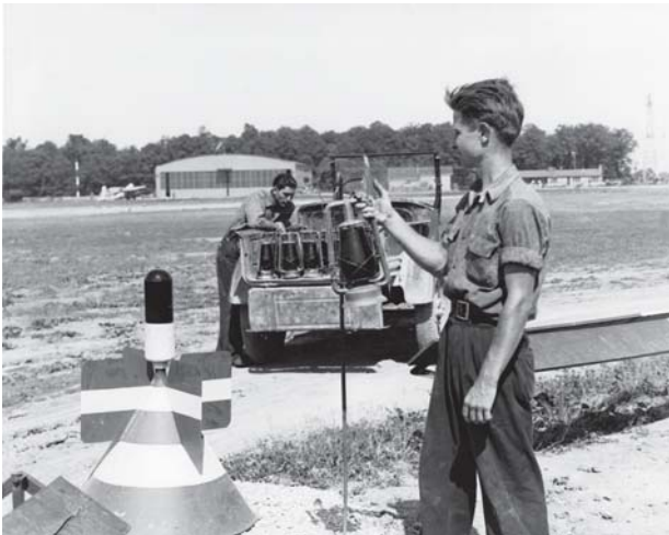
Electric lights replaced kerosene lanterns in 1936 to mark the boundaries of Paul Baer Municipal Airport. (Author's collection)
