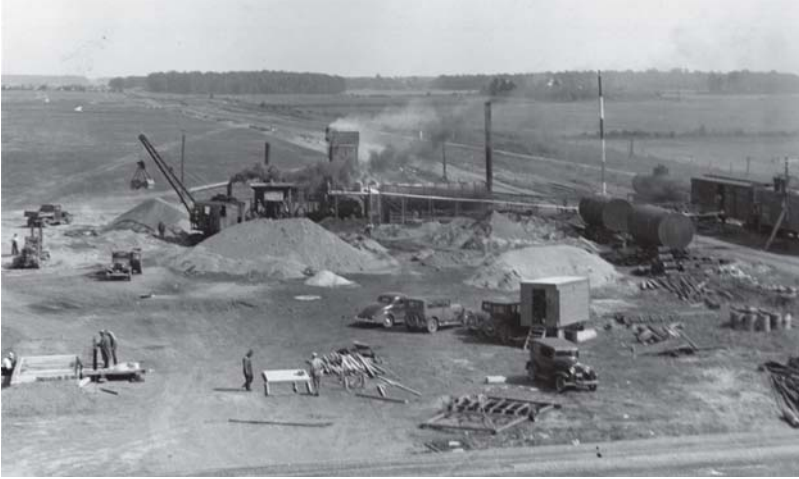
The asphalt used to pave Baer's runways was manufactured on site. (Author's collection)
