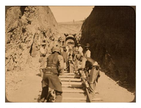
**Figure 47:** Photo of workers for Bachstein and Koppel laying the train line for the Nord-Südbahn through the Auas mountains. $^{76}$
