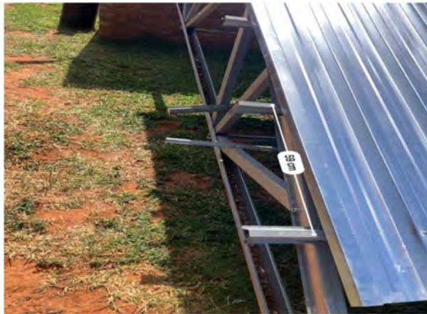
Figure 2. Showing the purlins spacing on the roof truss.
