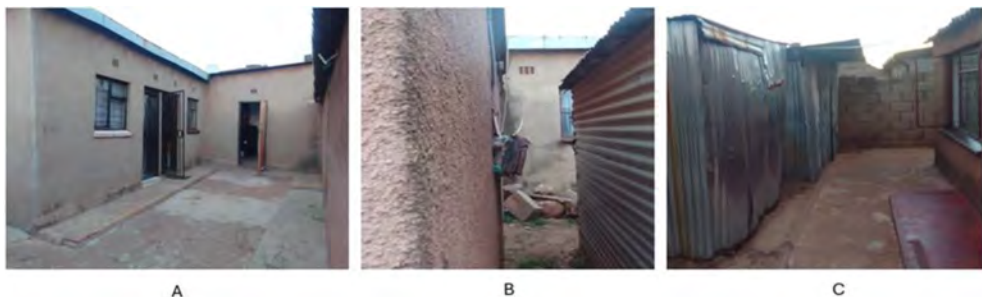
Figure 2. Electrification of backyard units (Author 2023).
