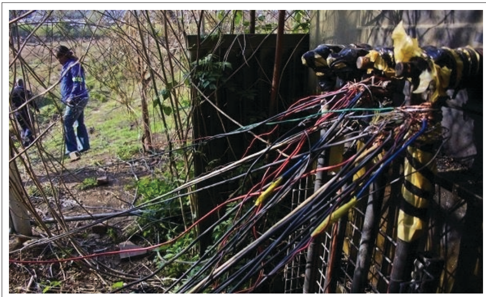
FIGURE 11.2: Photograph of hazardous illegal electricity supply connections.
