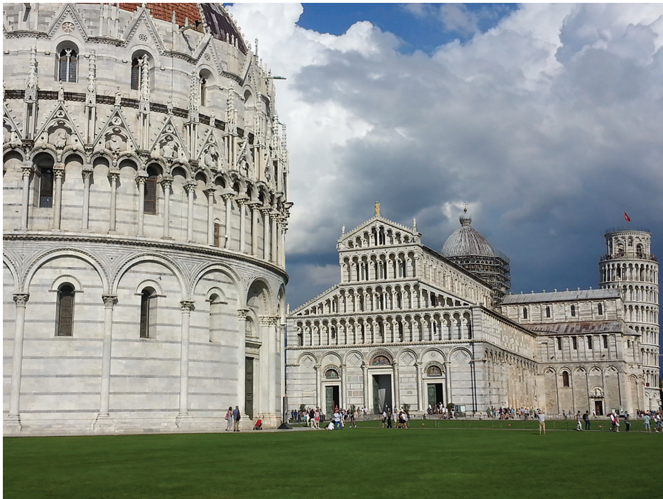
Figure 6.20 Pisa baptistery, cathedral, and bell tower, with blind arches surrounding the buildings at the bottom register, and arches with freestanding columns on the upper registers. Photo: author.
