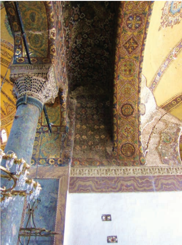
Figure 8.9 South gallery, eastern lateral arch, mosaics. Photo: author.
