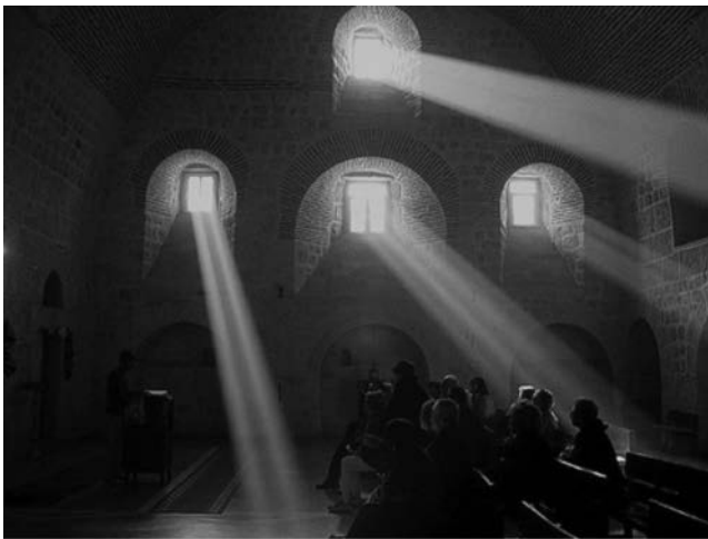
Figure 4.21 Light shafts through windows that widen toward the interior. Dayro d-Mor Gabriel (The Monastery of Saint Gabriel), 4th century, Tur Abdin plateau, near Midyat town, Mardin Province, Southeastern Turkey. Photo: author.
