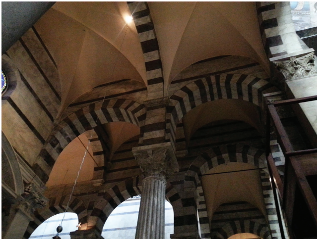
Figure 6.15 View of the intersection between south aisles and transept, Pisa cathedral. The multiple arches with black and white voussoirs spanning out of single columns and pillars create the visual impression of fanning palm trees. Photo: author.
