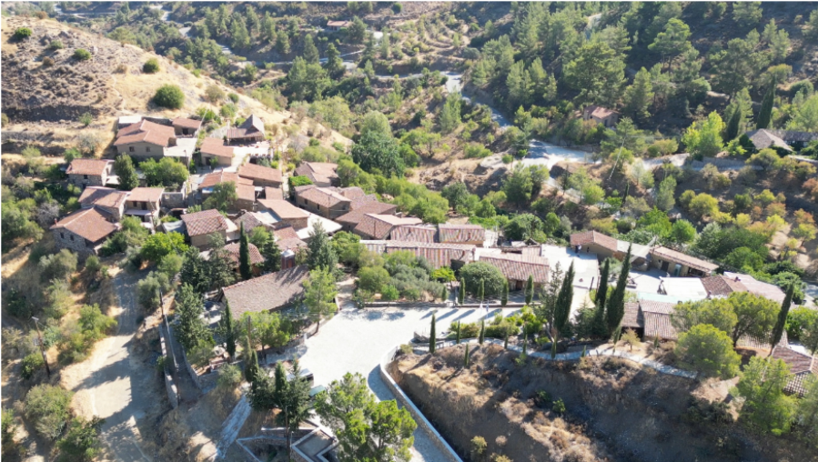
Fig. 4. Drone Image, overview of the Fikardou village
