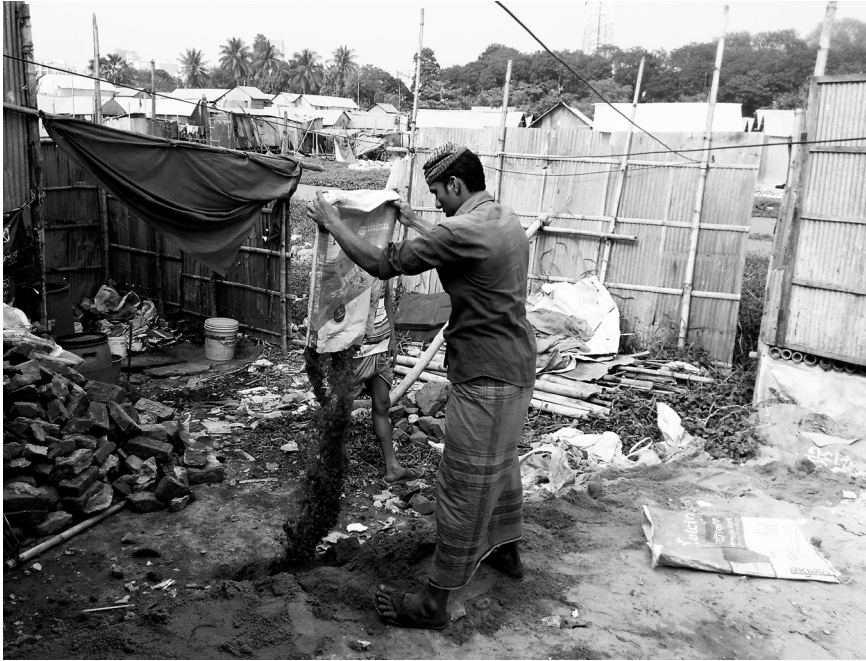
Figure 17 Filling up the lake to make new land!
