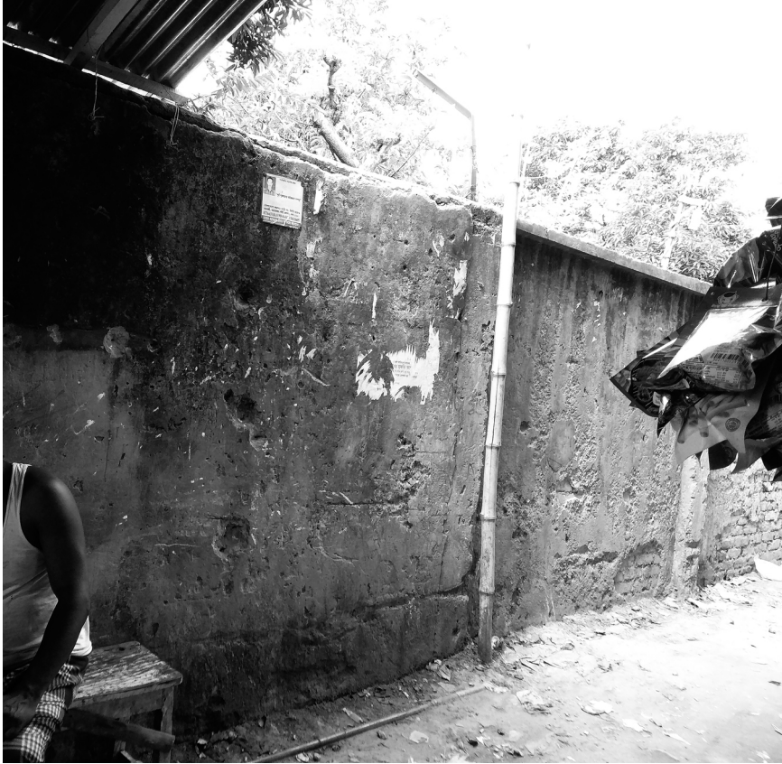
Figure 6 The wall was built with double the original thickness in this particular spot.
