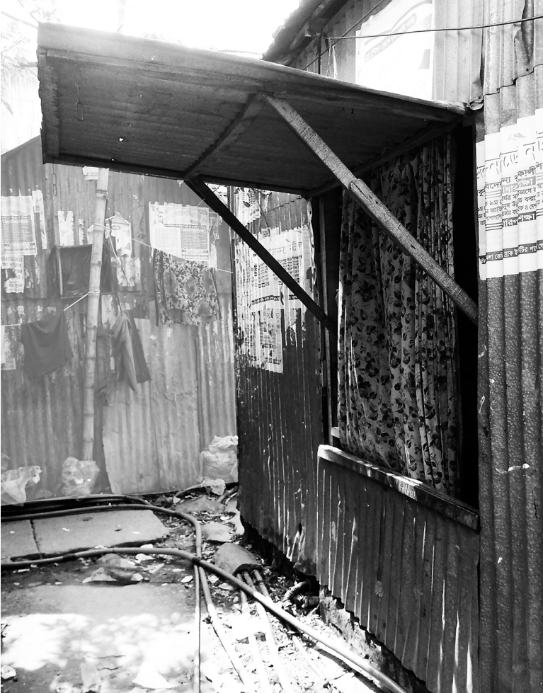
Figure 30 The dwelling unit converted to a tailoring shop by just cutting a window.
