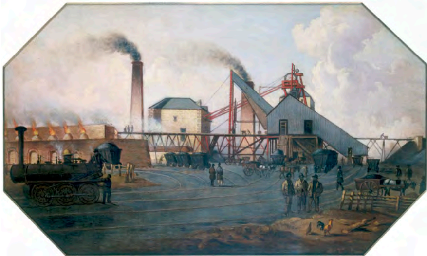
6.6 The original 'beehive' coke ovens at Pease's West colliery are shown on the left of this painting, W. Wheldon, 'North Eastern coalfield: colliery pit-head and coking ovens in England'. (c. 1845). Source: Science Museum Group Collection, ref. co521755.
