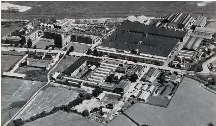
6.15 The expanded SEG site at Cheadle Heath (c. 1954). Source: Steam Power Plant , Simon-Carves Ltd (1955).
