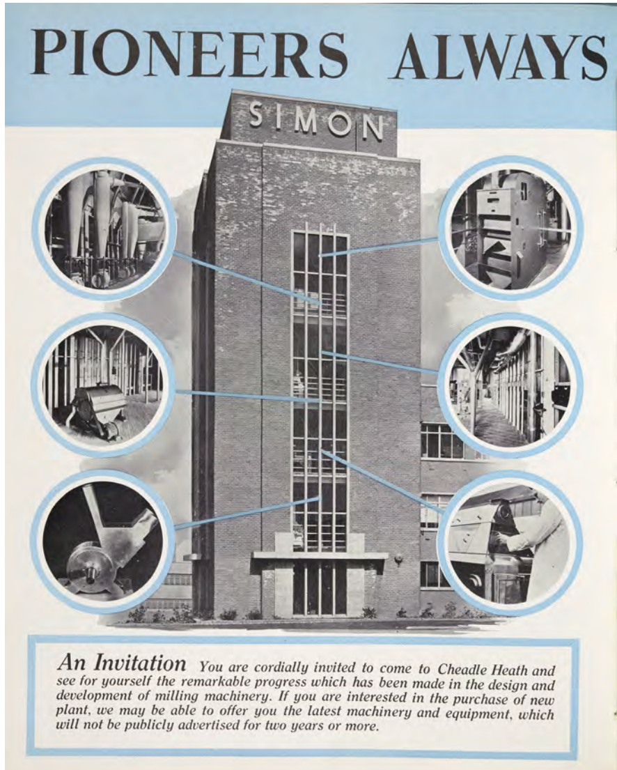
6.16 The tower containing a working model flour mill at Cheadle Heath topped off by a prominent 'SIMON' sign. Source: JRL SEGA, 23, Occasional Letter, 225, June 1953, p. 3. Copyright the University of Manchester (CC BY-NC-SA 4.0).
