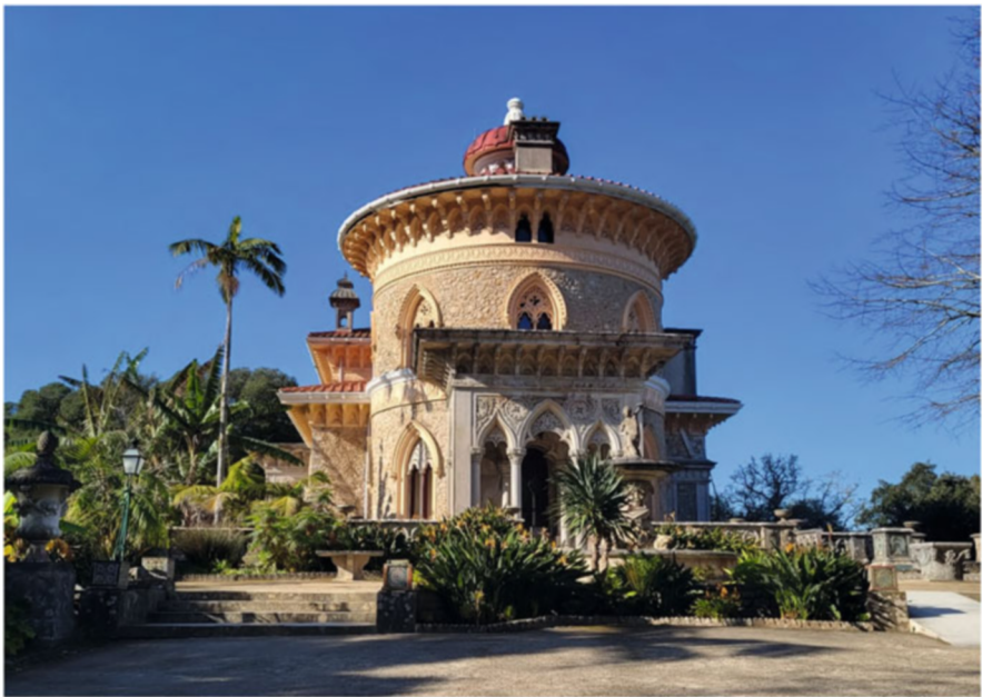
Fig. 13.1 Monserrate Palace entrance
