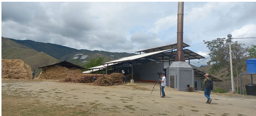
Fig. 11.6 View of the community sugar mill ( Trapiche Asociativo ) and bagasse from the cane used as fuel. (Photo: Castaño 2022)
