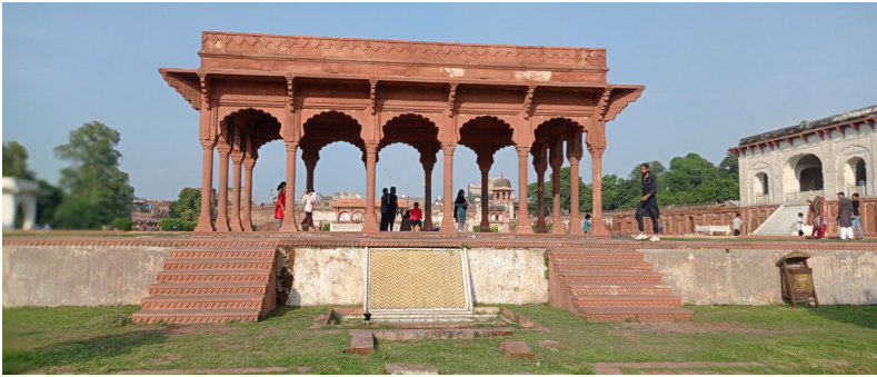
Figure 6.10 View of the Red Pavilion, western side, 2023. Image by Sajjad Kausar.
