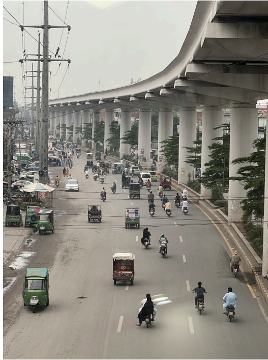
Figure 0.1 The Orange Line viaduct, 2022. Image by Hala Bashir Malik.
