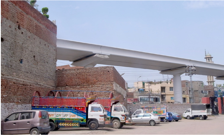
Figure 18.1 The Orange Line's elevated track, photographed from Evernew Studios, 2018. Image by Timothy P. A. Cooper.
