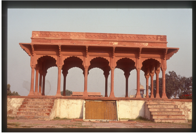
Figure 6.9 View of the Red Pavilion, western side, 1986. Image by Sajjad Kausar.
